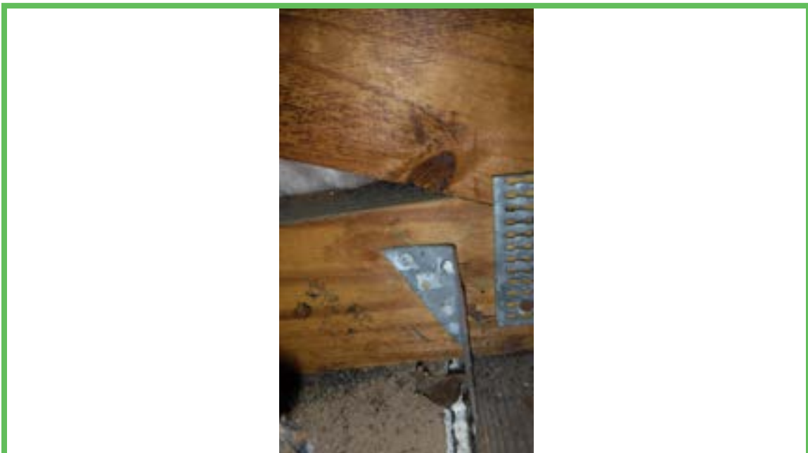
Roof to Wall Attachment
