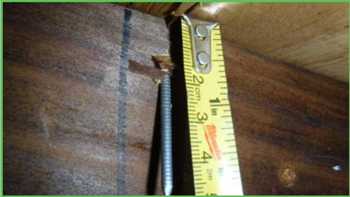
Roof Deck Attachment
