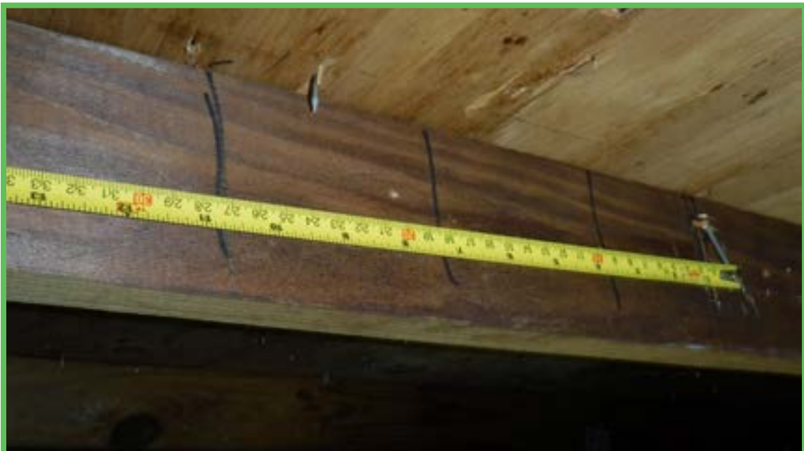
Roof Deck Attachment
