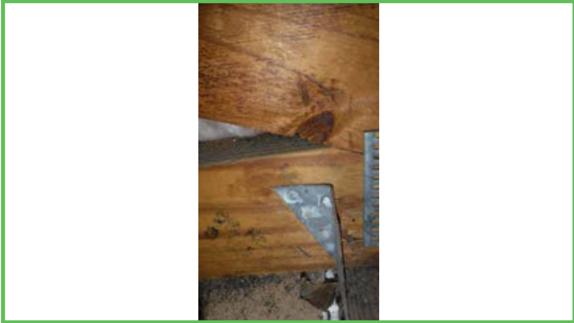
Roof to Wall Attachment
