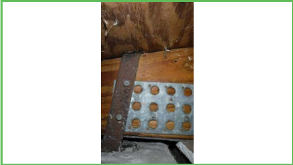
Roof to Wall Attachment
