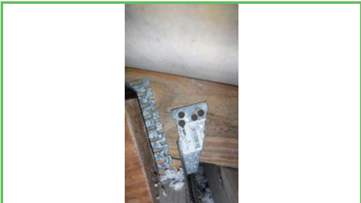
Roof to Wall Attachment
