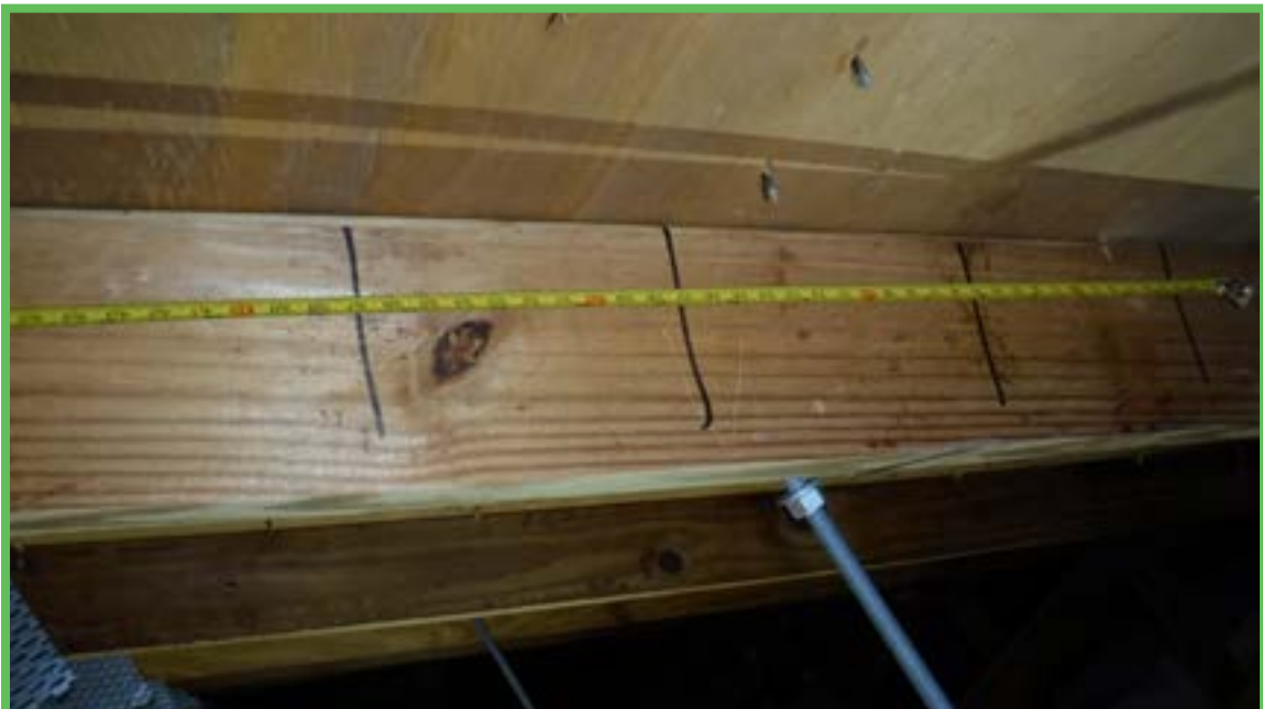
Roof Deck Attachment
