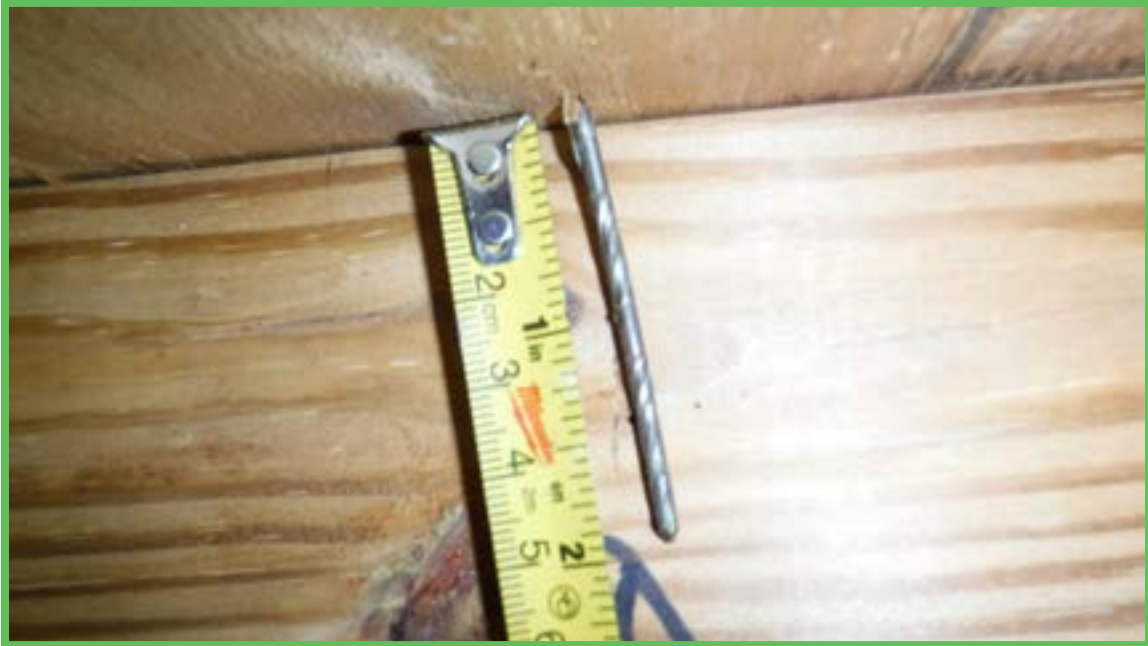
Roof Deck Attachment
