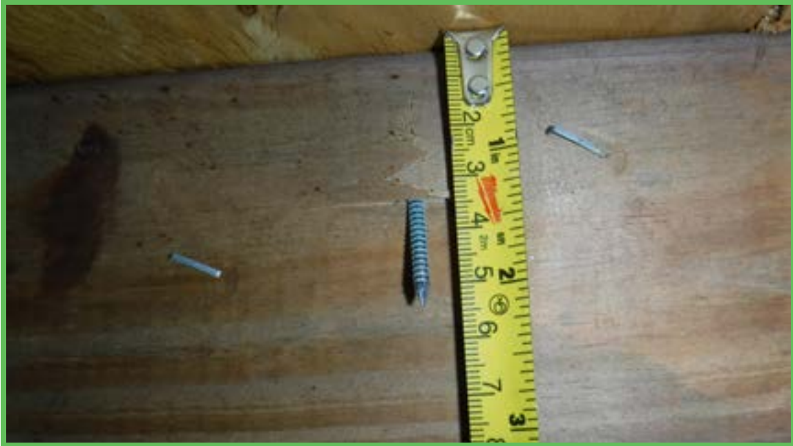
Roof Deck Attachment
