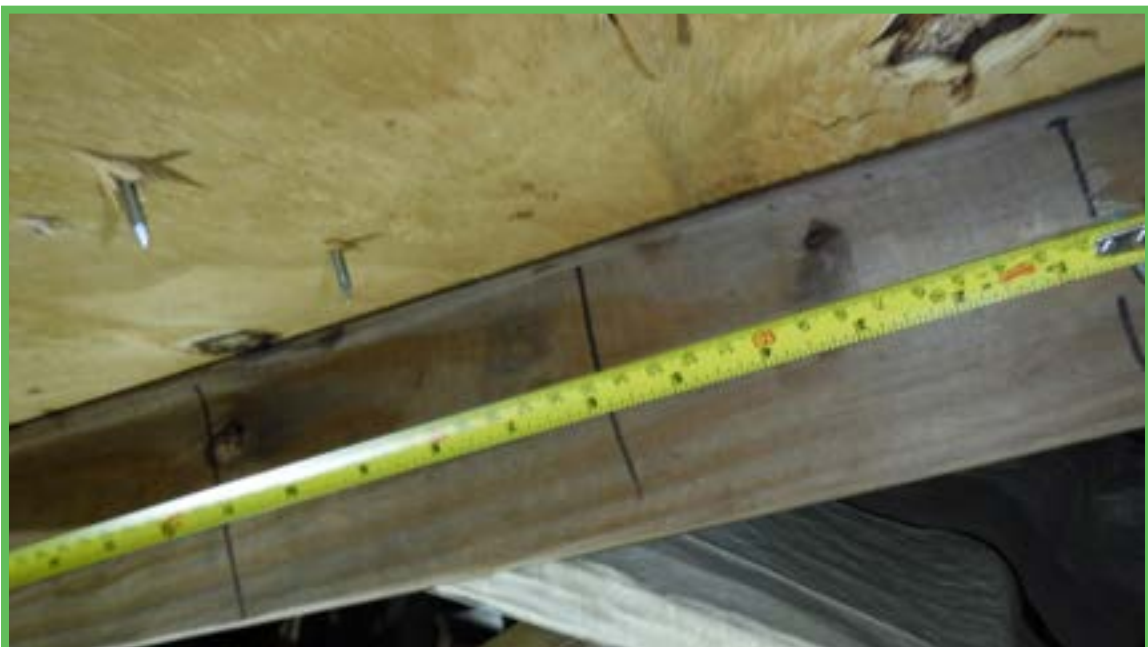
Roof Deck Attachment
