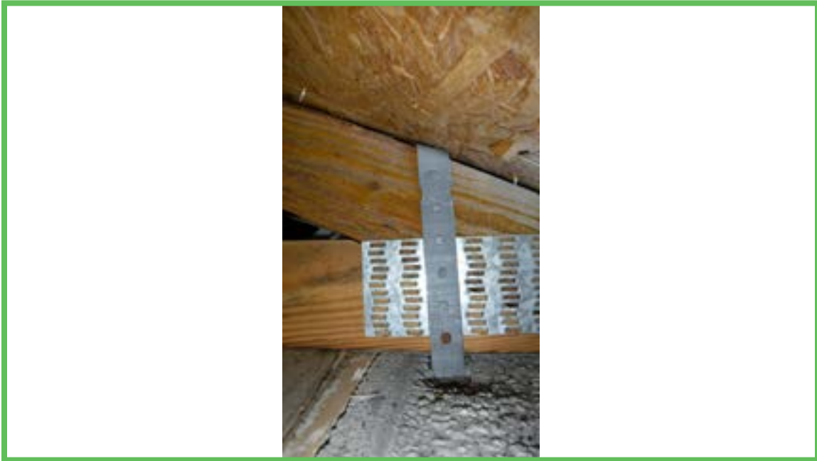
Roof to Wall Attachment
