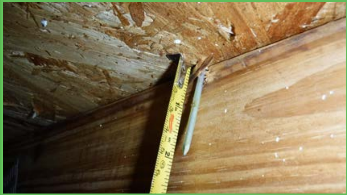
Roof Deck Attachment
