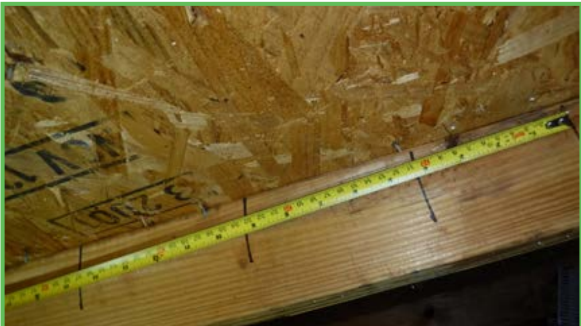
Roof Deck Attachment
