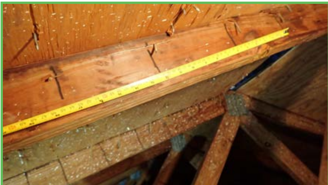
Roof Deck Attachment
