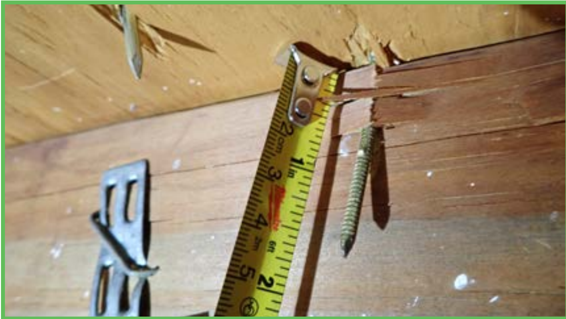
Roof Deck Attachment
