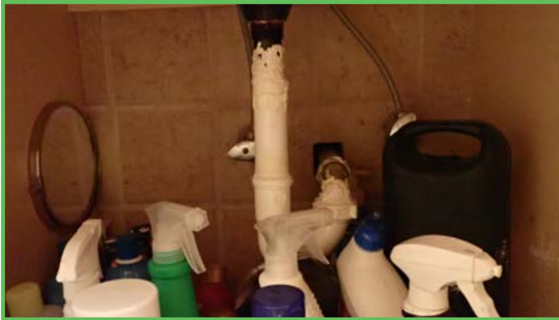
Under Sink1 Bath 1
