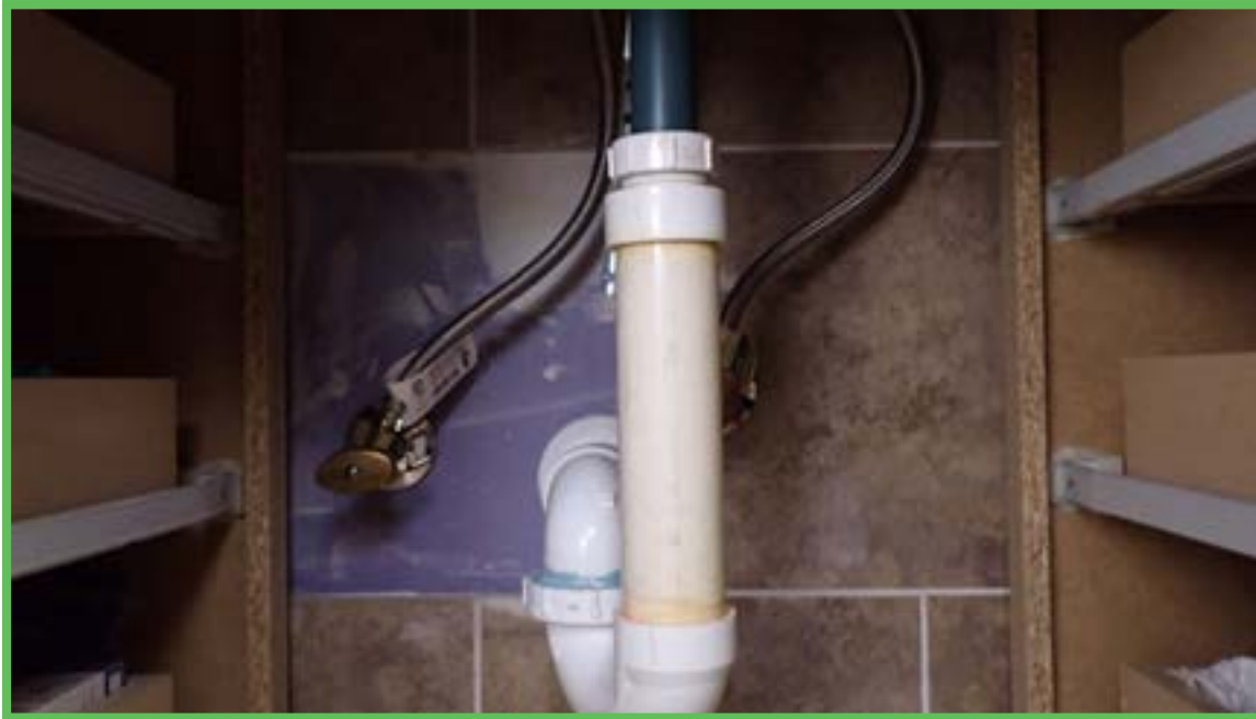
Under Sink1 Bath 2
