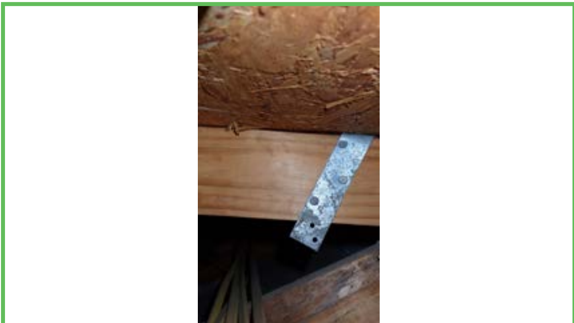
Roof to Wall Attachment
