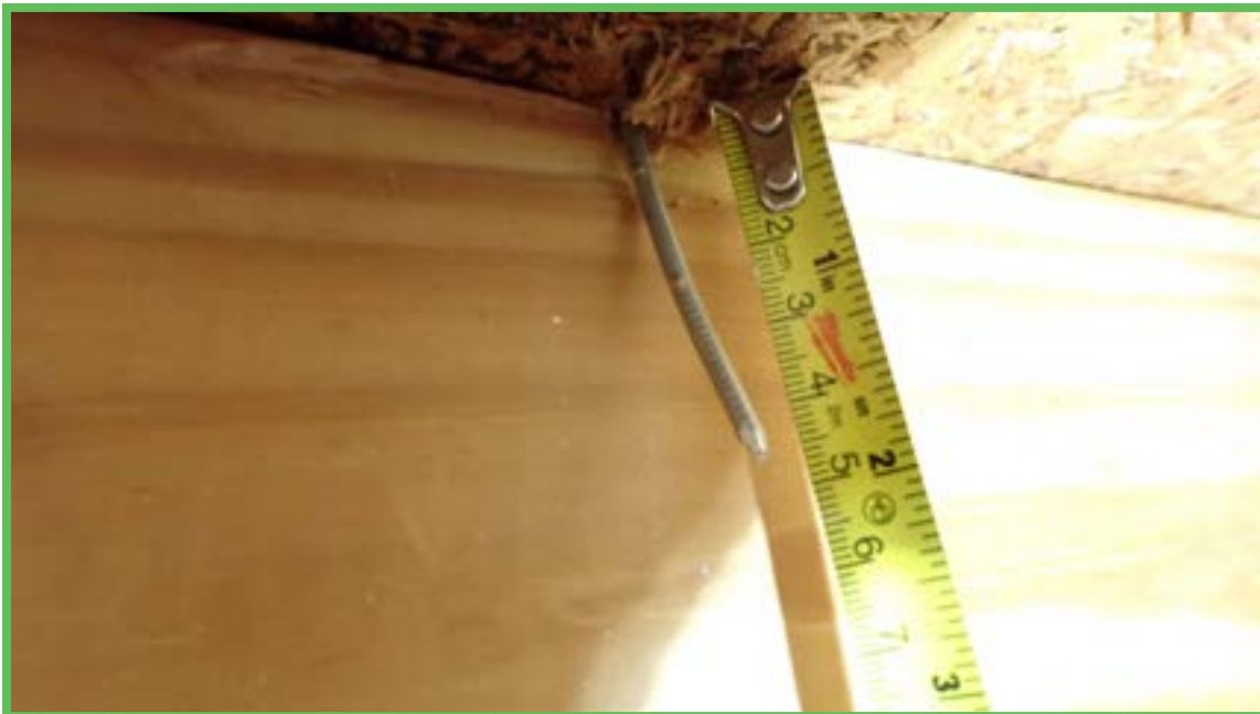
Roof Deck Attachment
