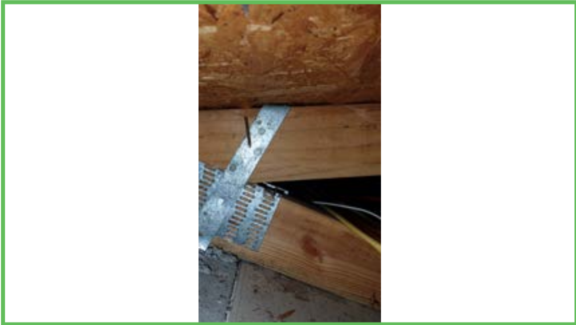
Roof to Wall Attachment
