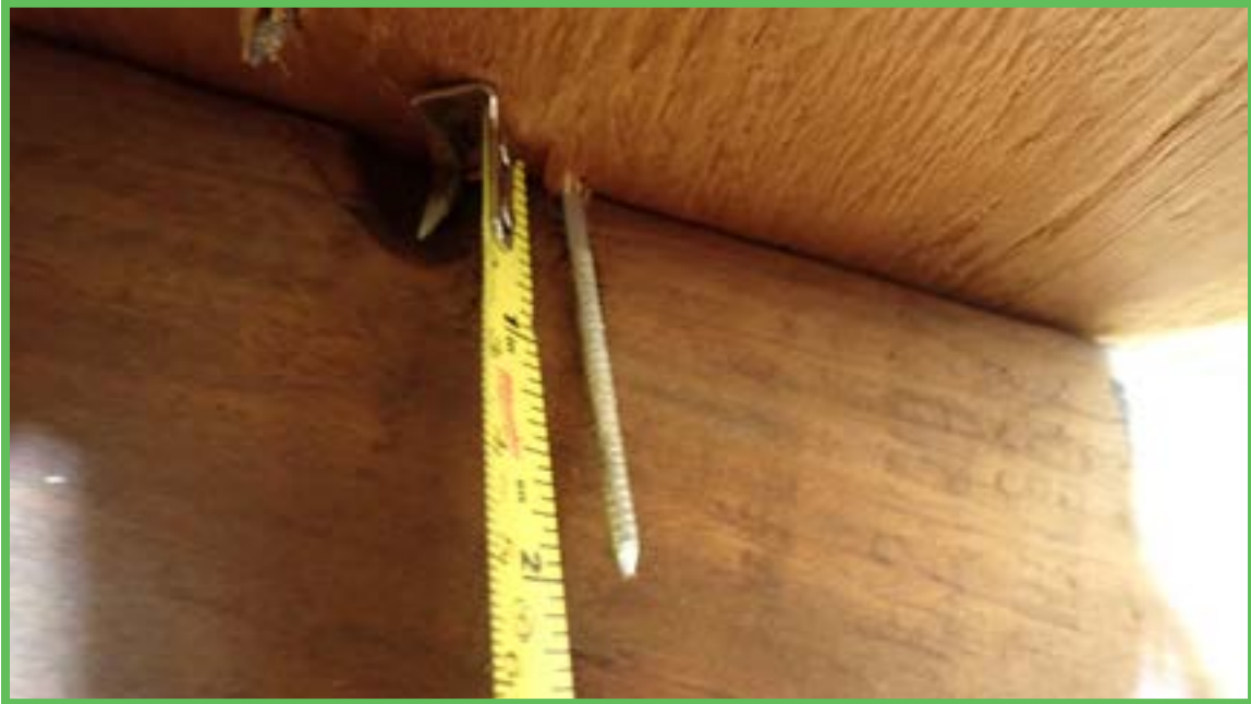
Roof Deck Attachment
