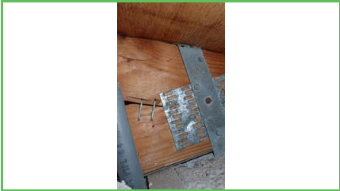
Roof to Wall Attachment
