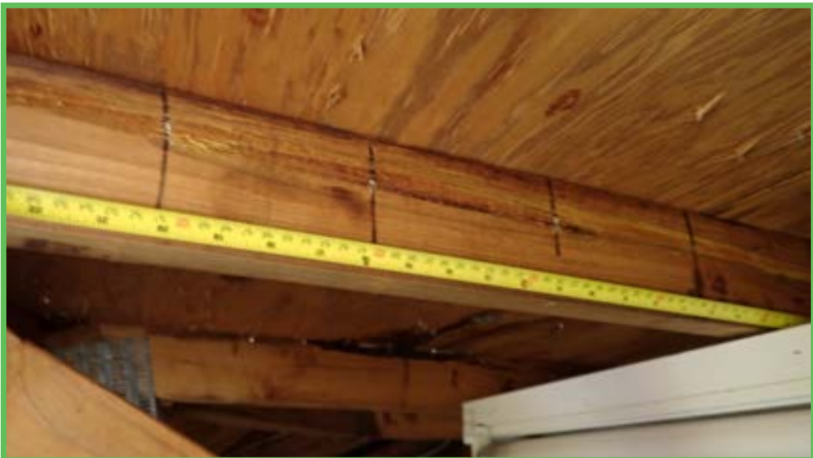
Roof Deck Attachment
