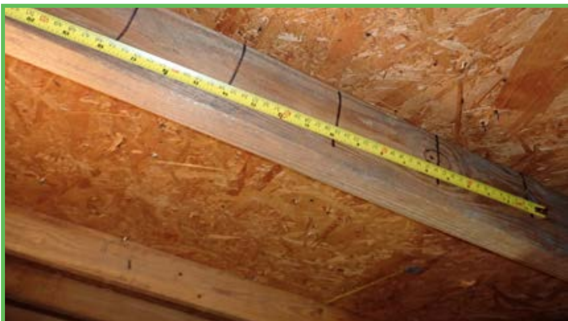
Roof Deck Attachment
