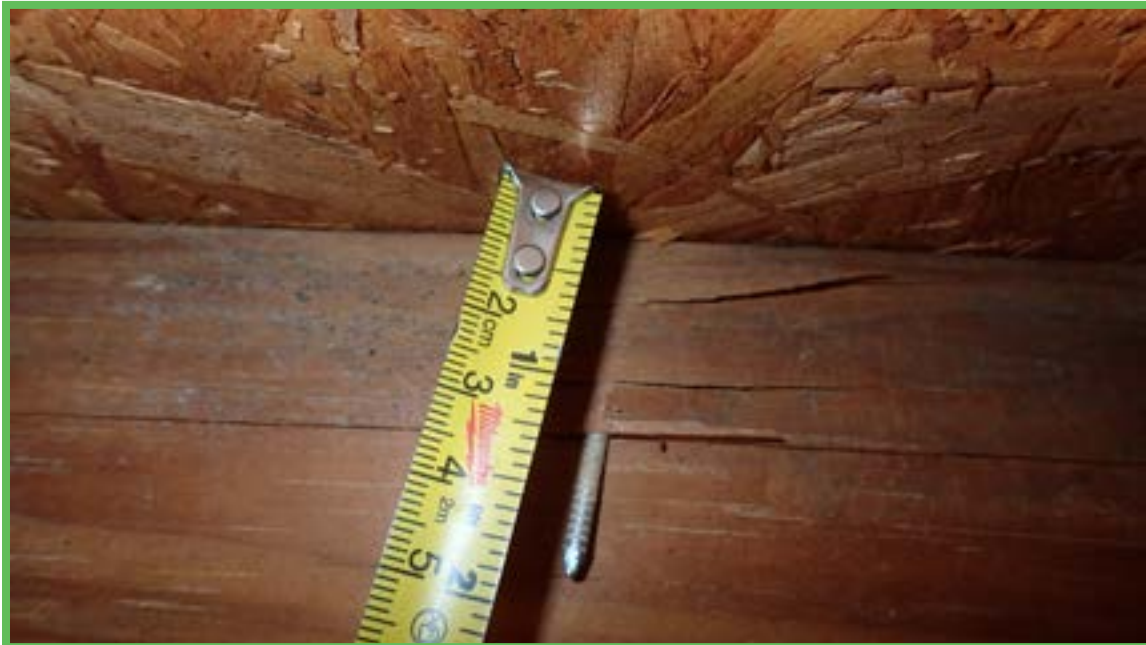
Roof Deck Attachment
