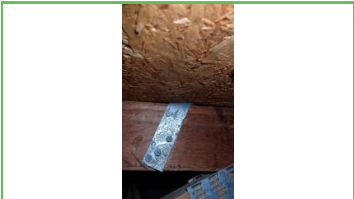
Roof to Wall Attachment
