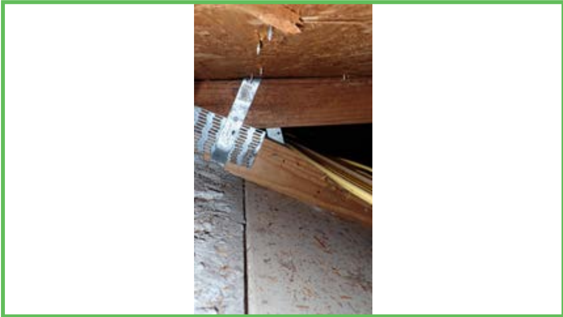
Roof to Wall Attachment
