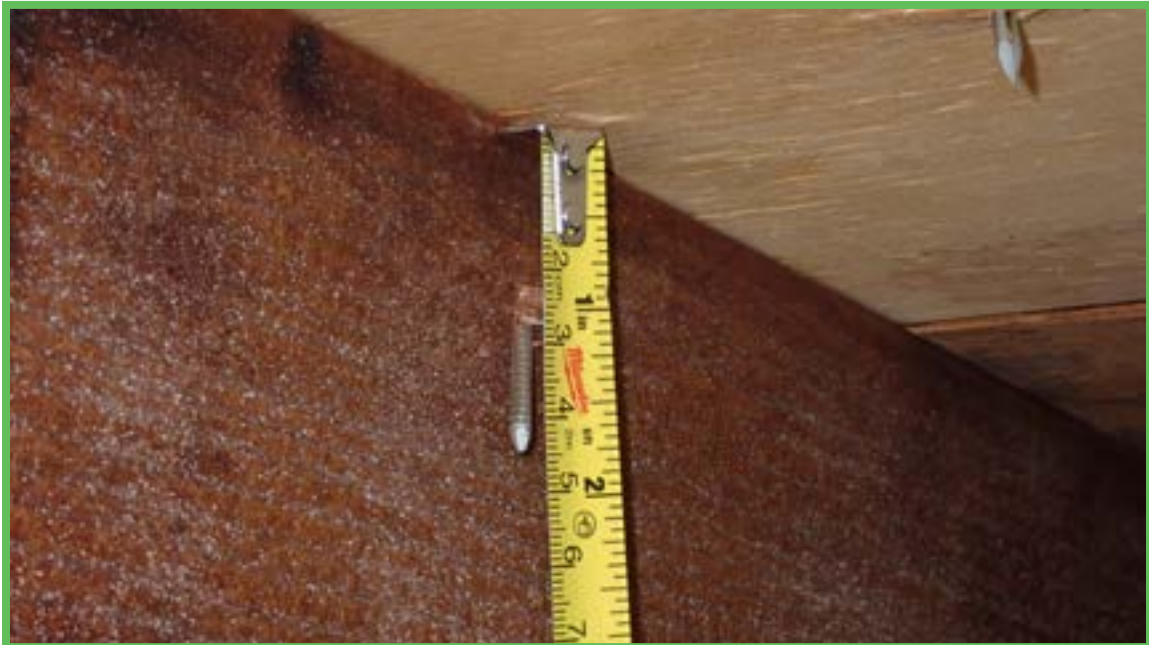
Roof Deck Attachment
