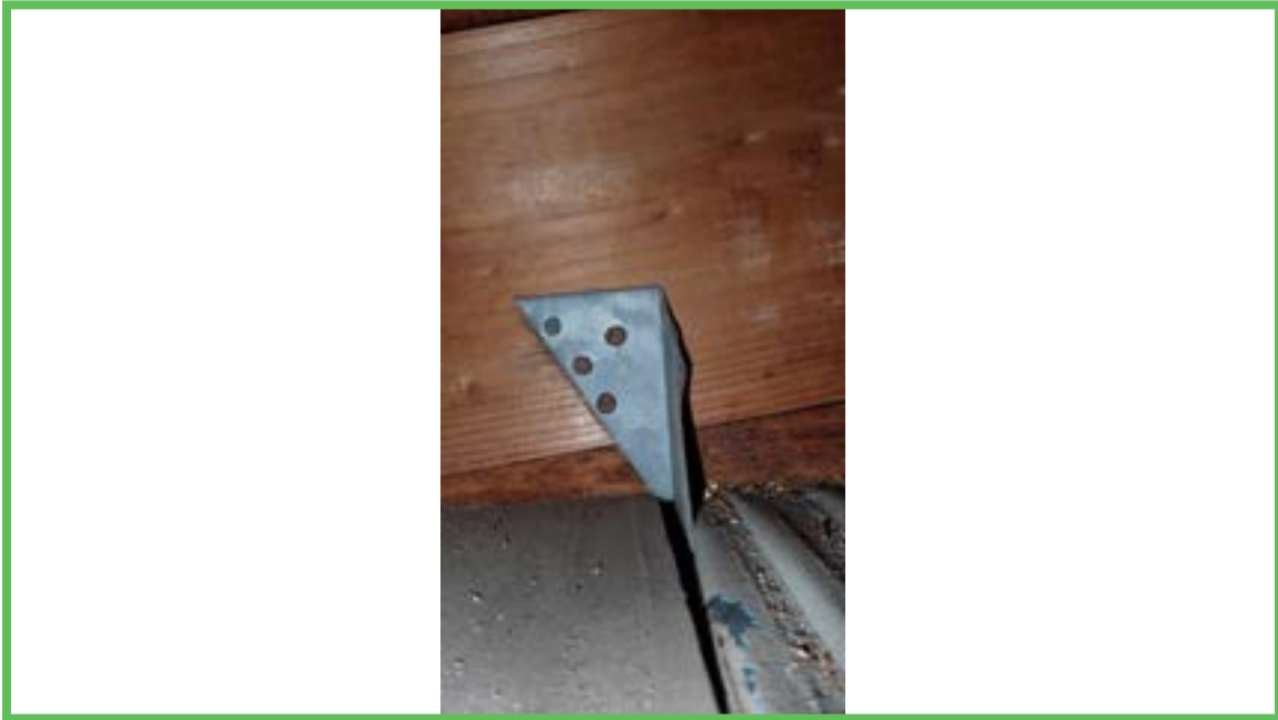
Roof to Wall Attachment
