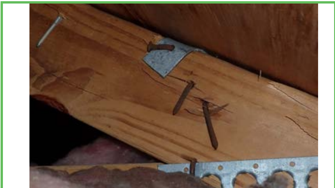
Roof to Wall Attachment
