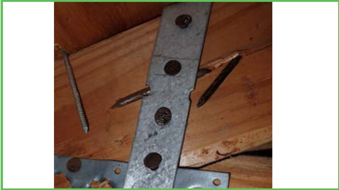
Roof to Wall Attachment
