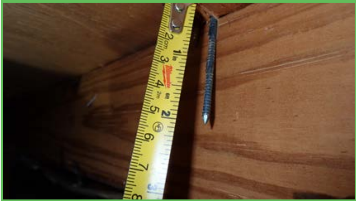
Roof Deck Attachment
