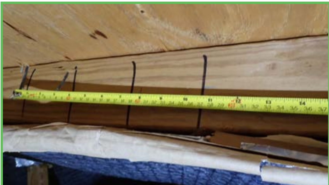
Roof Deck Attachment
