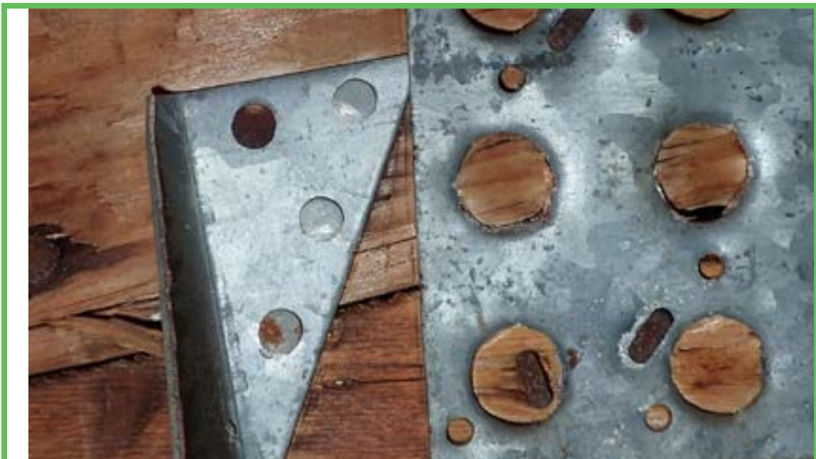
Roof to Wall Attachment
