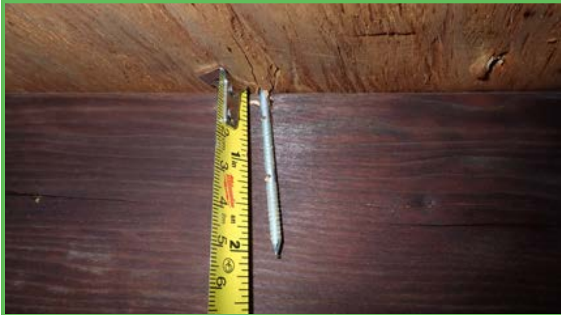
Roof Deck Attachment
