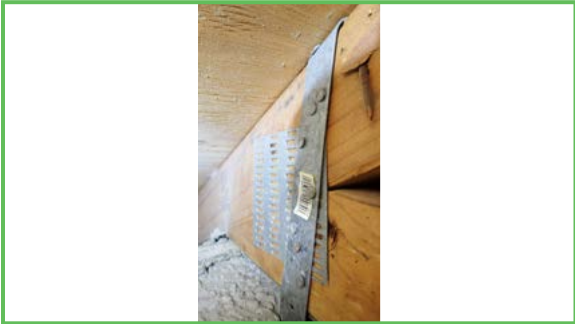
Roof to Wall Attachment
