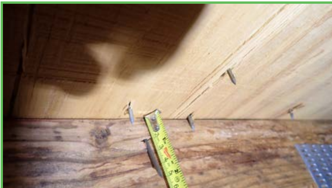
Roof Deck Attachment
