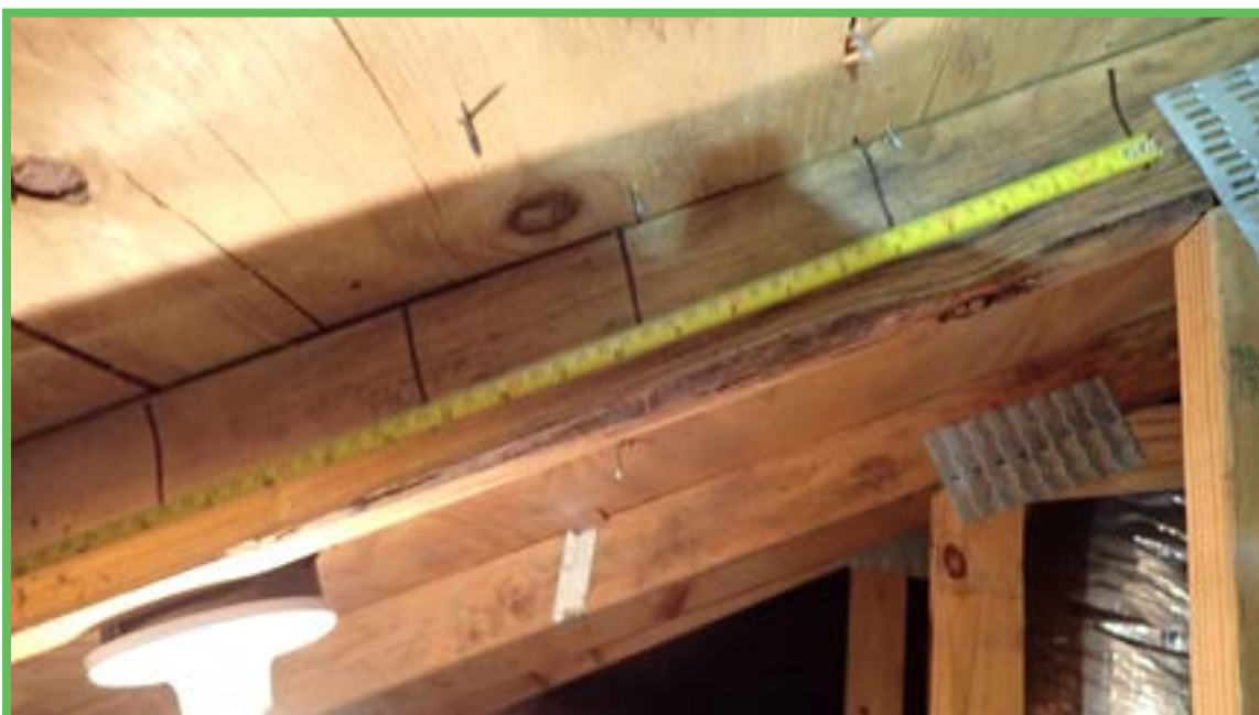
Roof Deck Attachment
