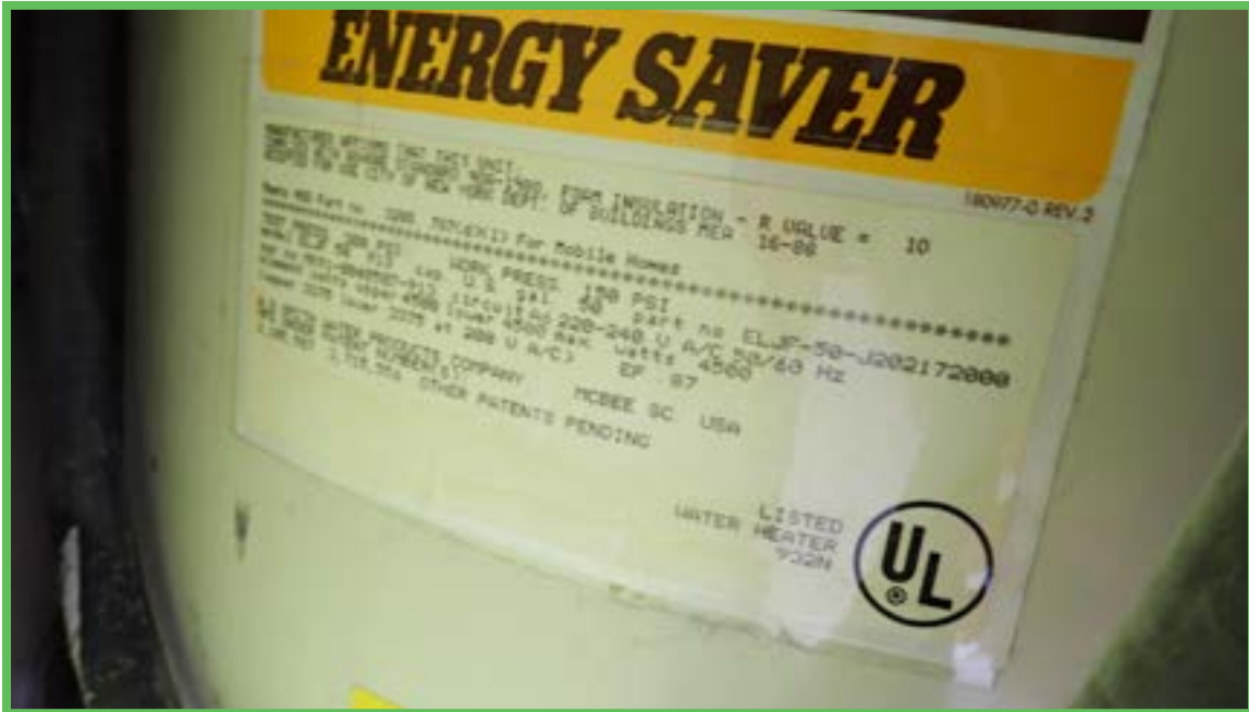
Water Heater Data Plate
