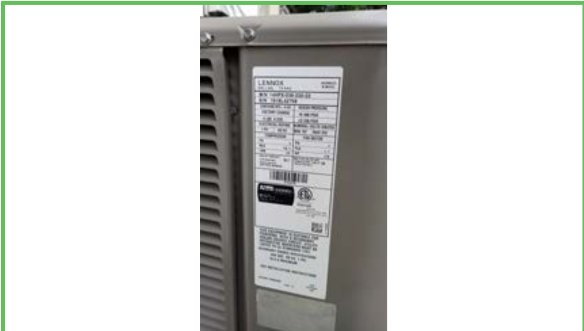
HVAC Condenser Data Plate
