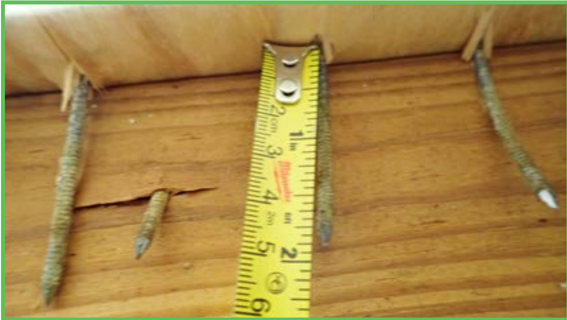
Roof Deck Attachment
