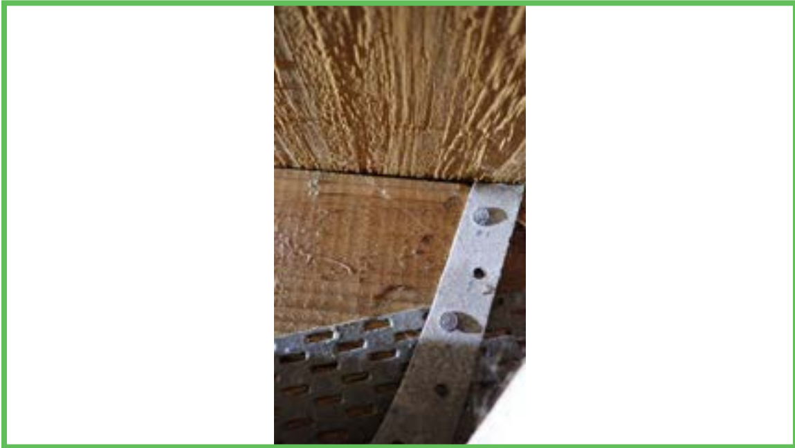
Roof to Wall Attachment
