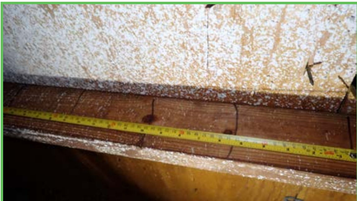
Roof Deck Attachment
