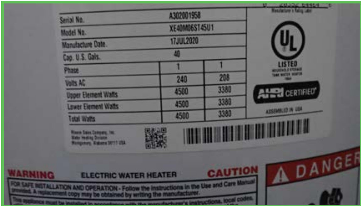
Water Heater Data Plate
