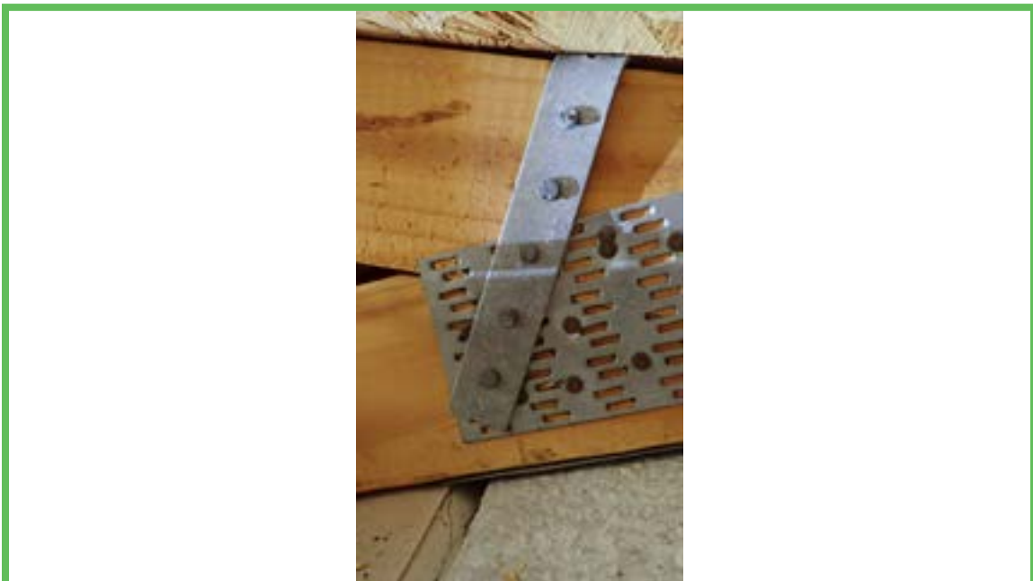
Roof to Wall Attachment
