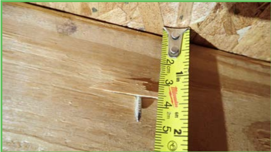
Roof Deck Attachment
