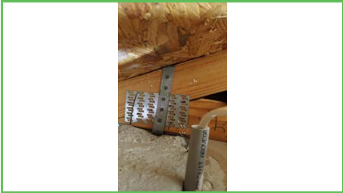
Roof to Wall Attachment
