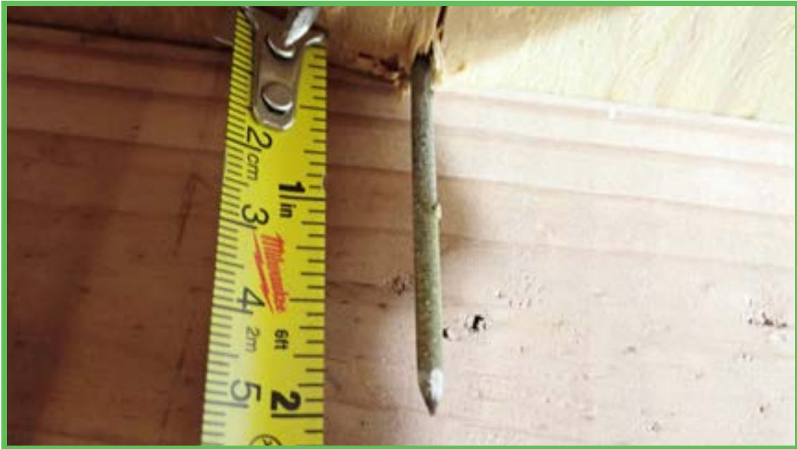
Roof Deck Attachment
