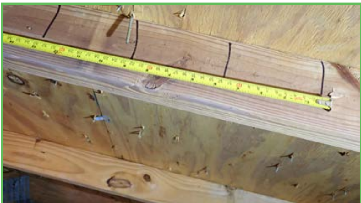
Roof Deck Attachment
