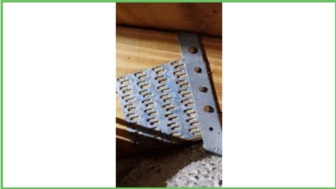
Roof to Wall Attachment
