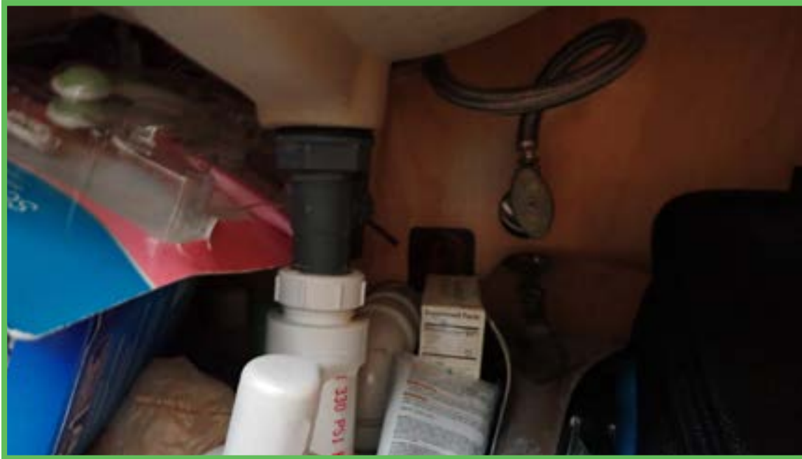
Under Sink1 Bath 1
