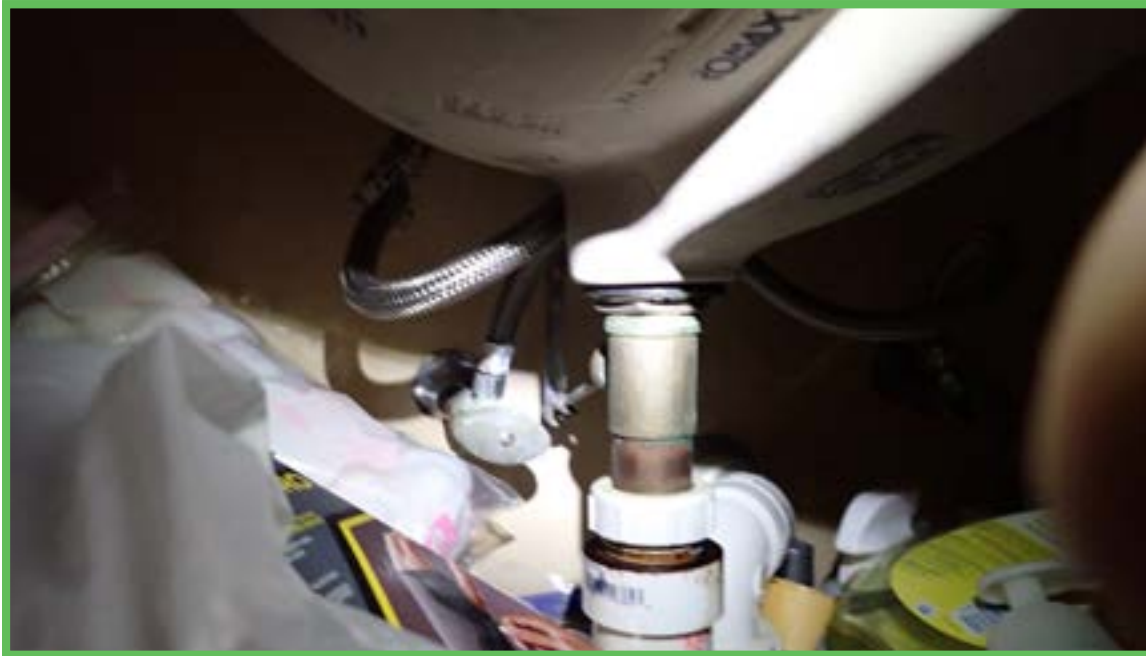
Under Sink1 Bath 2
