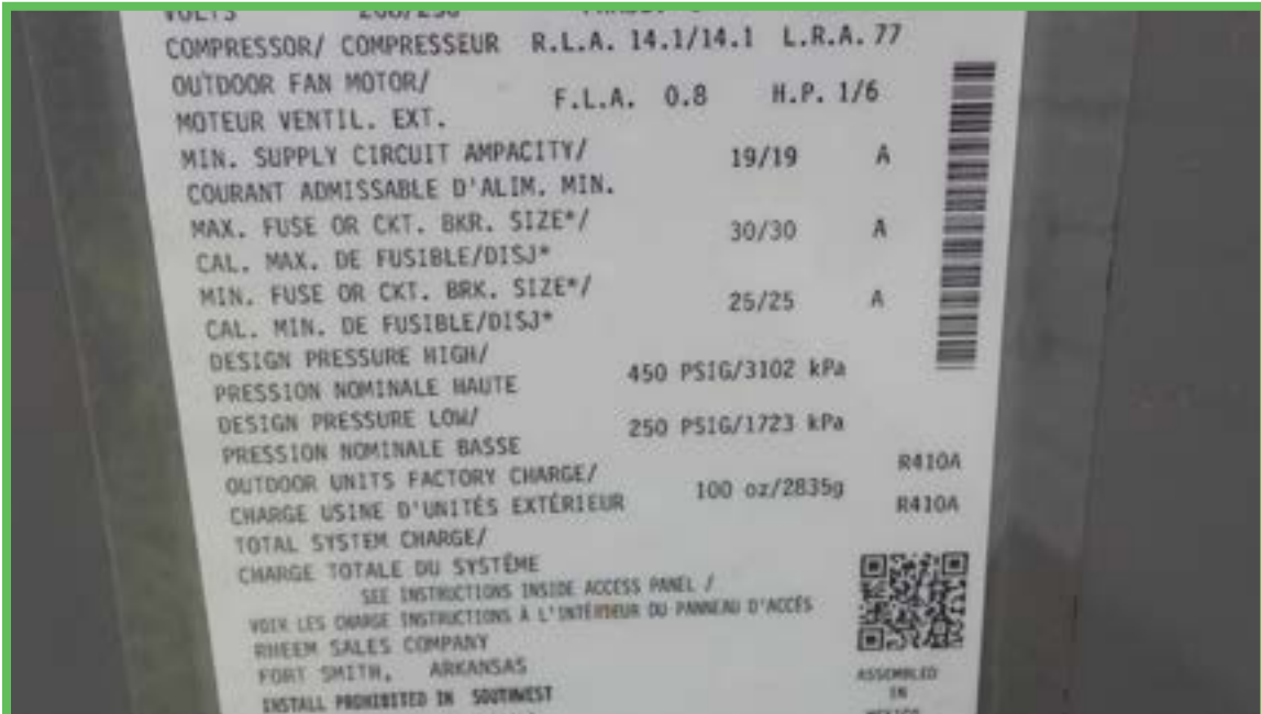
HVAC Condenser Data Plate
