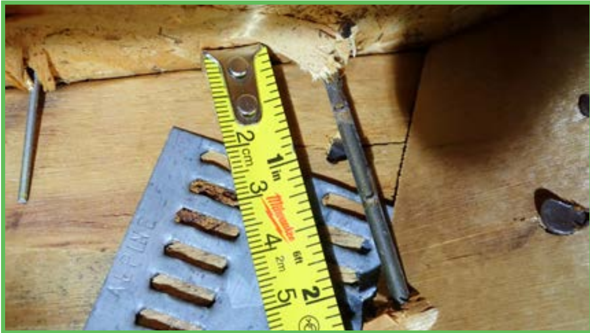
Roof Deck Attachment
