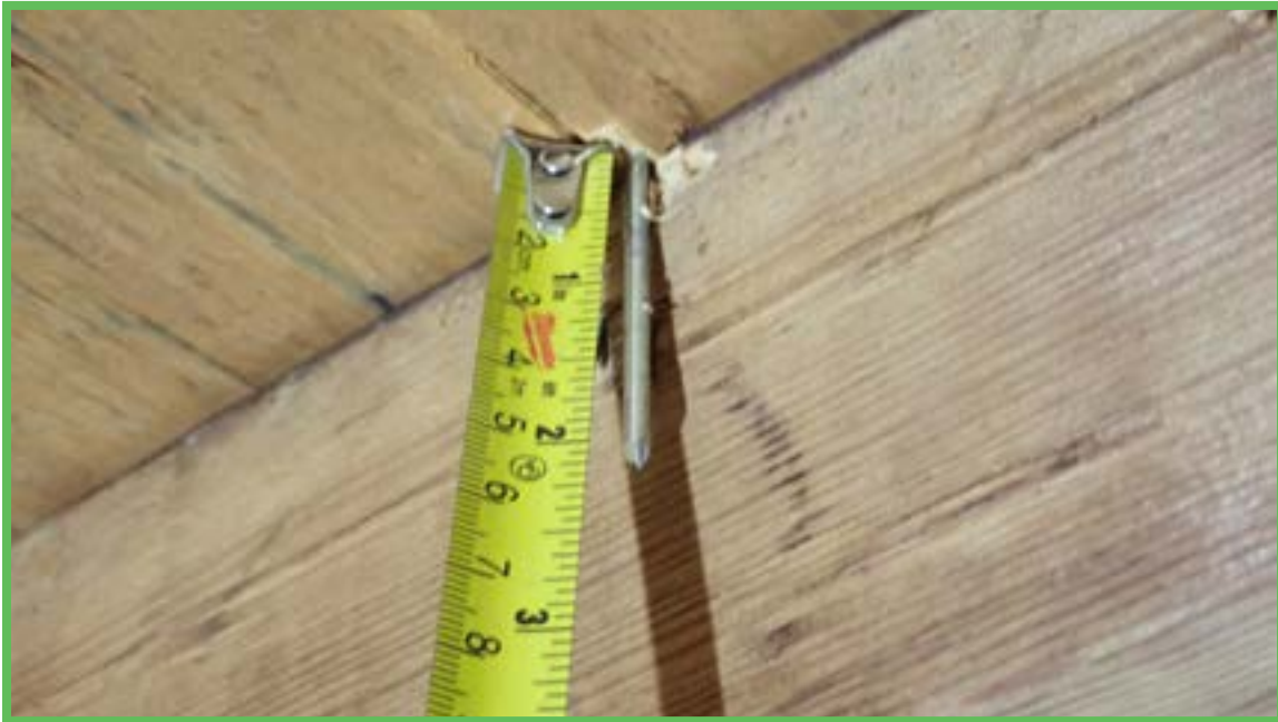
Roof Deck Attachment
