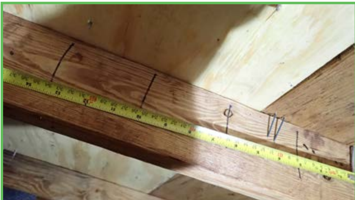
Roof Deck Attachment
