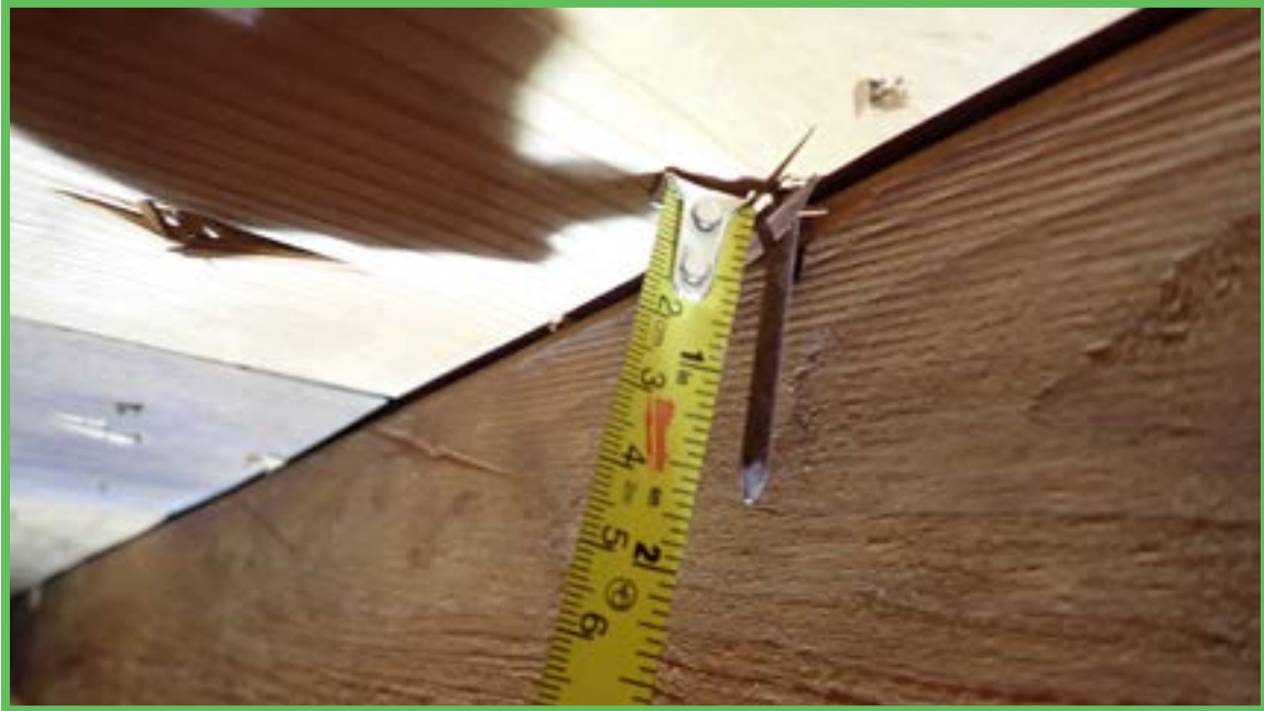
Roof Deck Attachment
