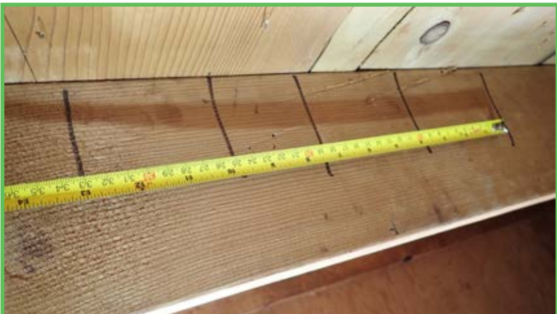
Roof Deck Attachment
