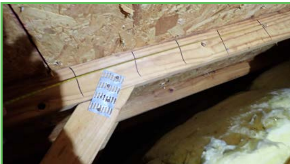
Roof Deck Attachment
