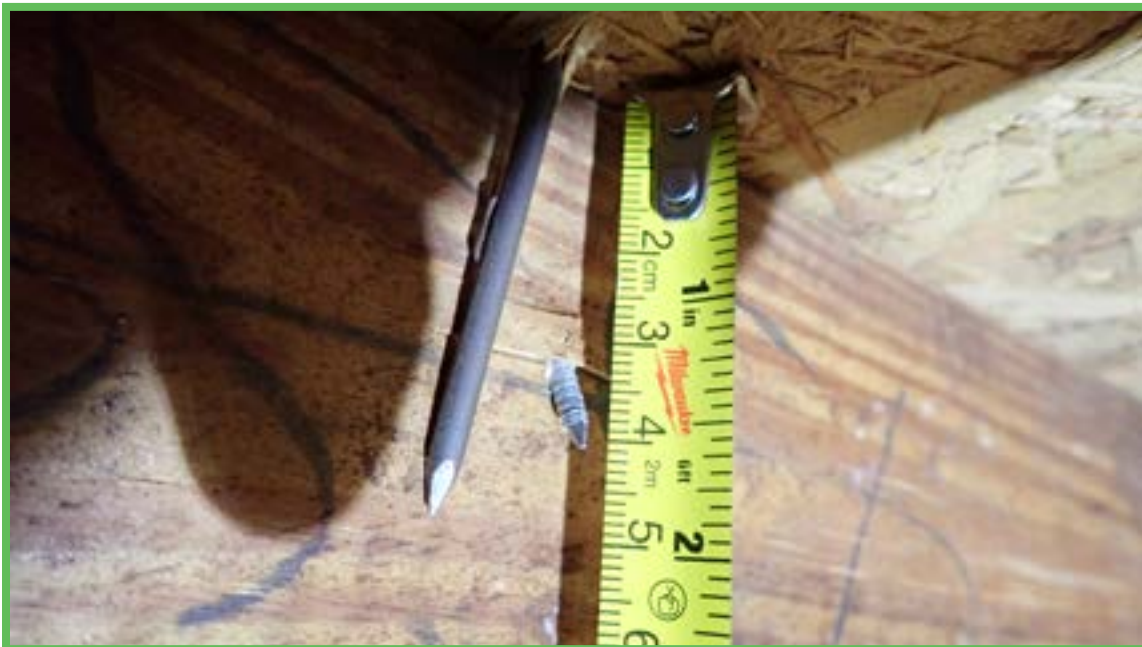
Roof Deck Attachment
