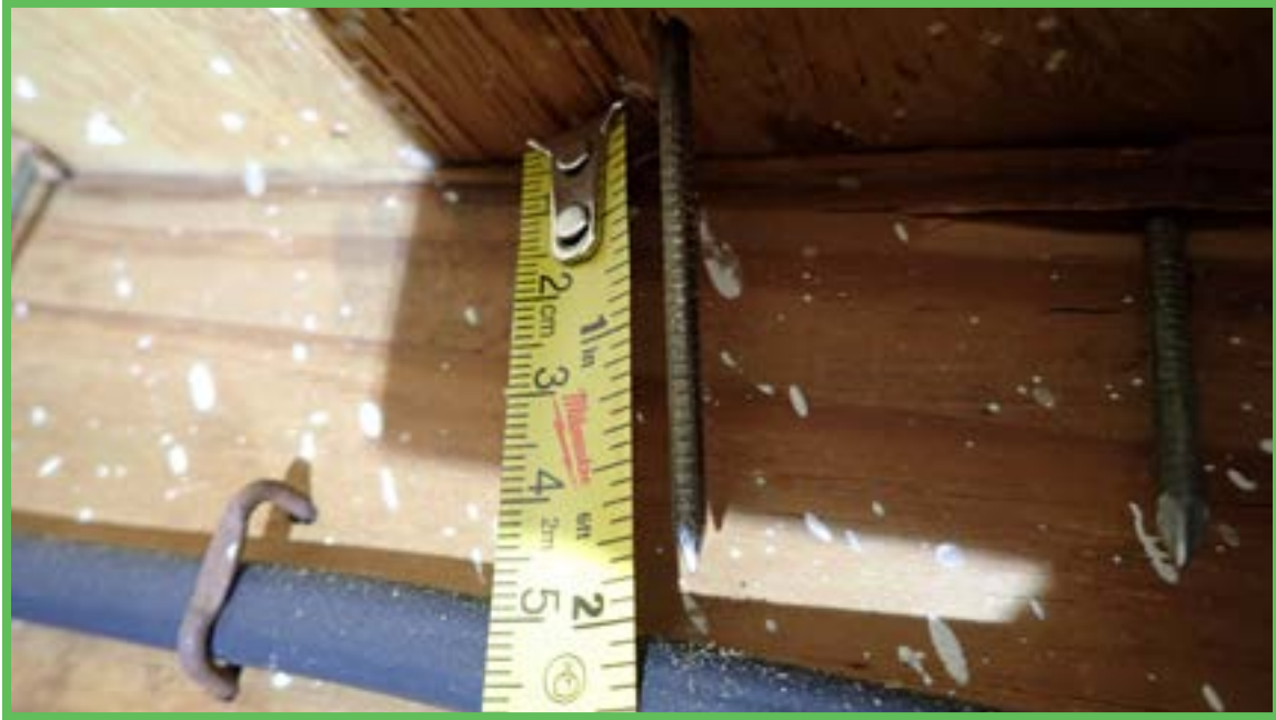
Roof Deck Attachment
