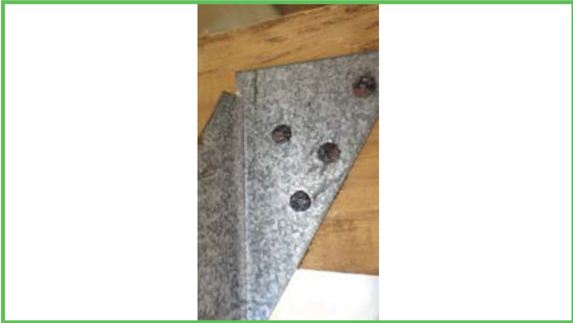
Roof to Wall Attachment
