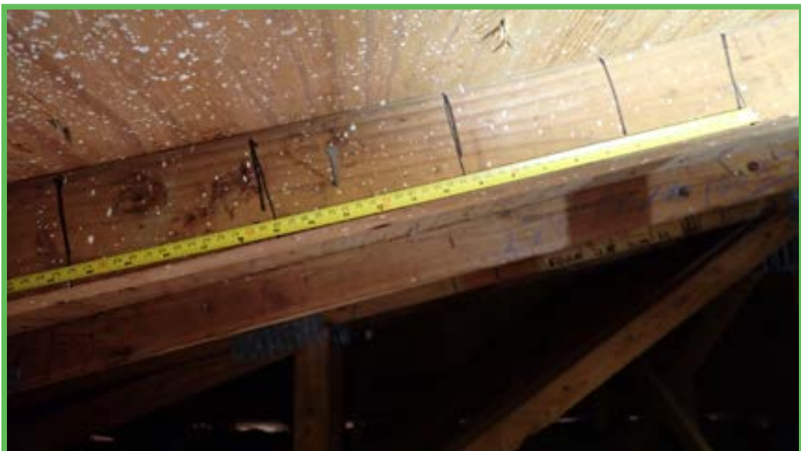
Roof Deck Attachment
