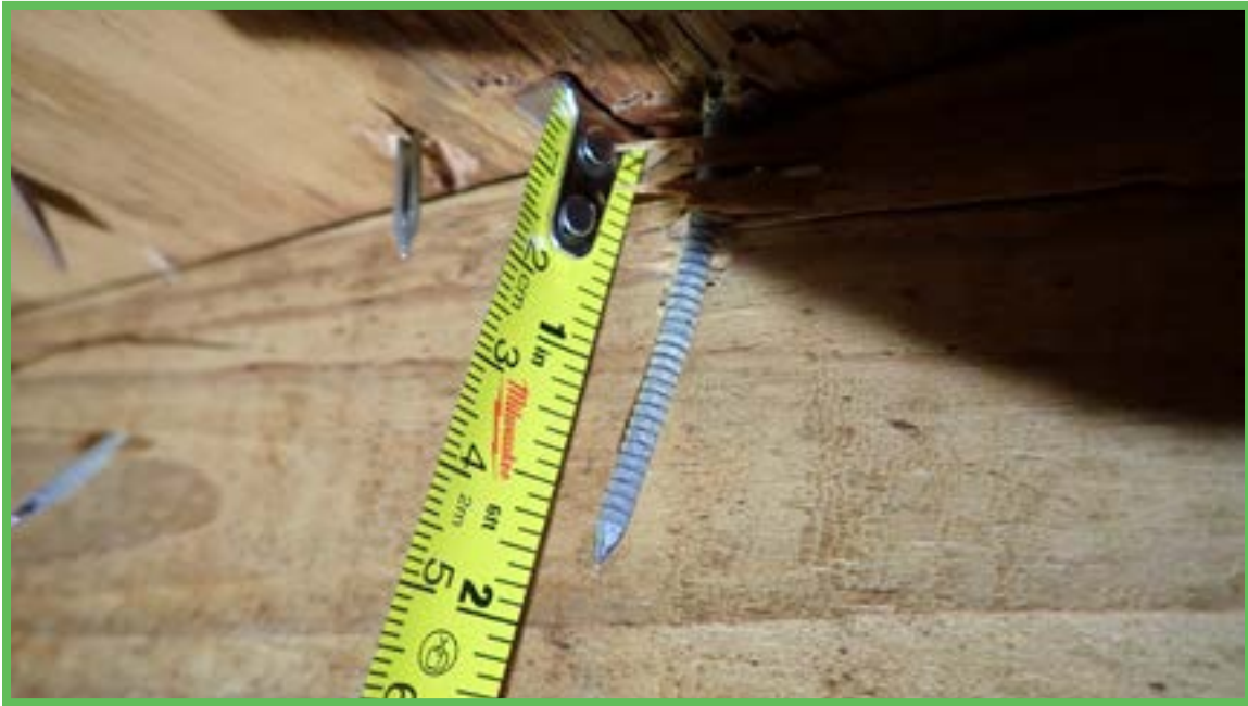
Roof Deck Attachment
