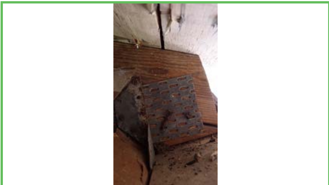
Roof to Wall Attachment
