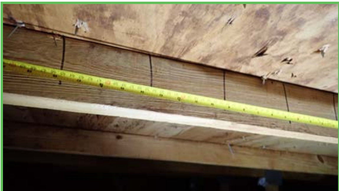
Roof Deck Attachment
