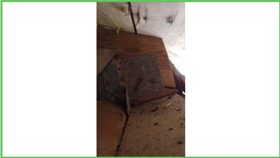
Roof to Wall Attachment
