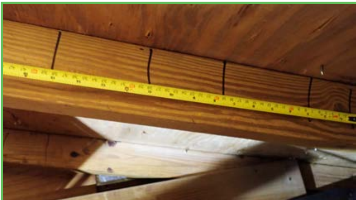
Roof Deck Attachment
