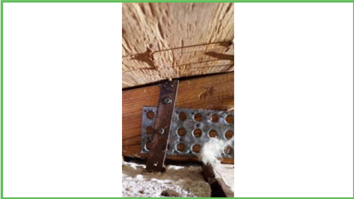
Roof to Wall Attachment
