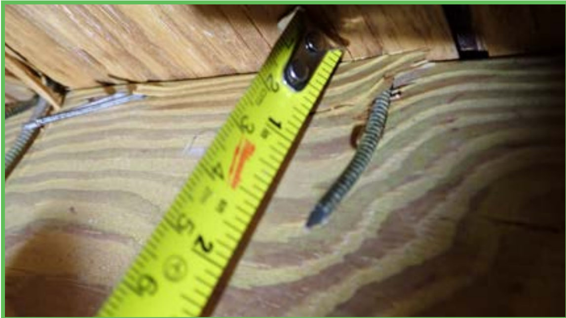
Roof Deck Attachment
