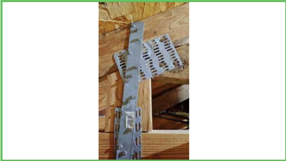
Roof to Wall Attachment
