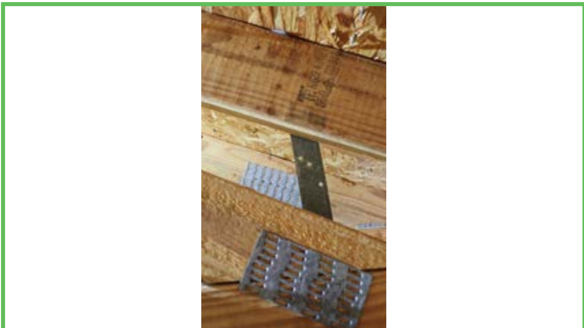
Roof to Wall Attachment
