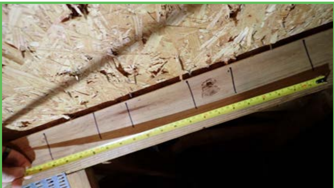
Roof Deck Attachment
