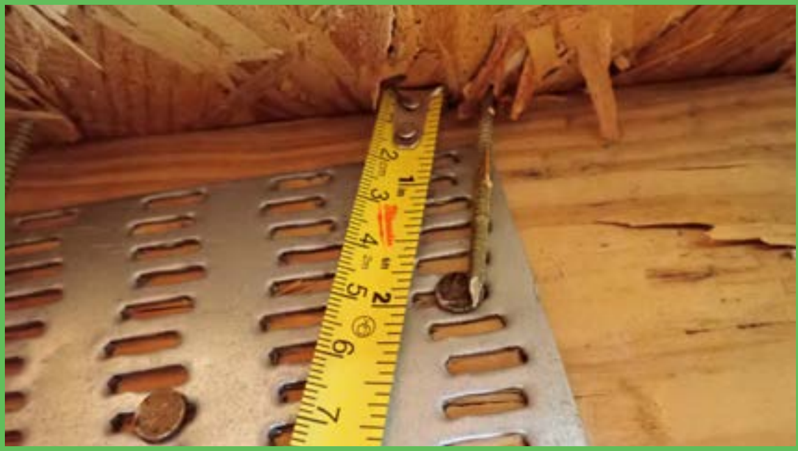
Roof Deck Attachment
