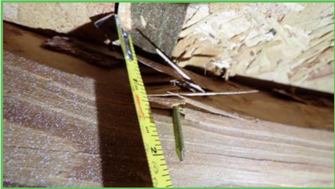
Roof Deck Attachment
