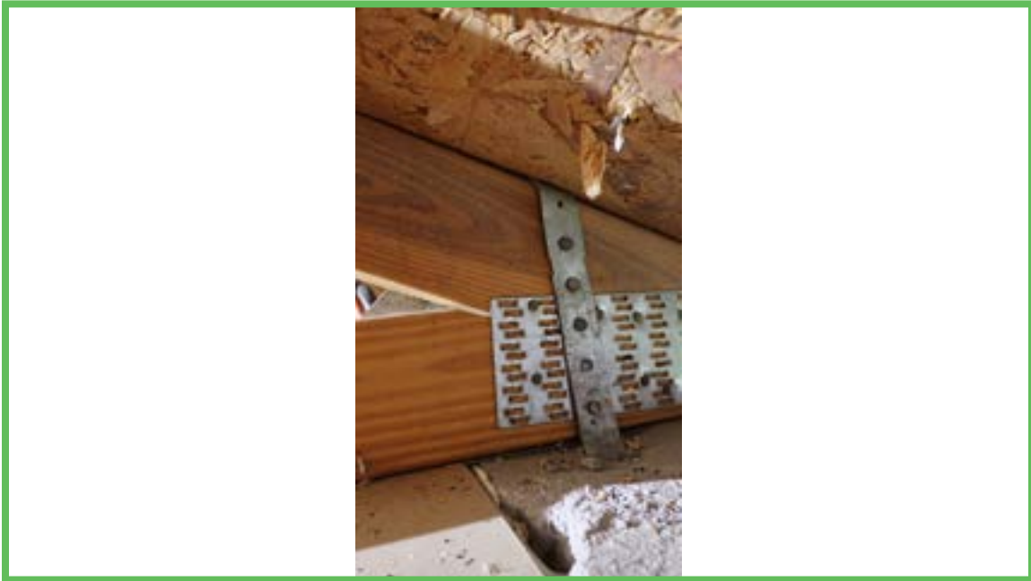
Roof to Wall Attachment
