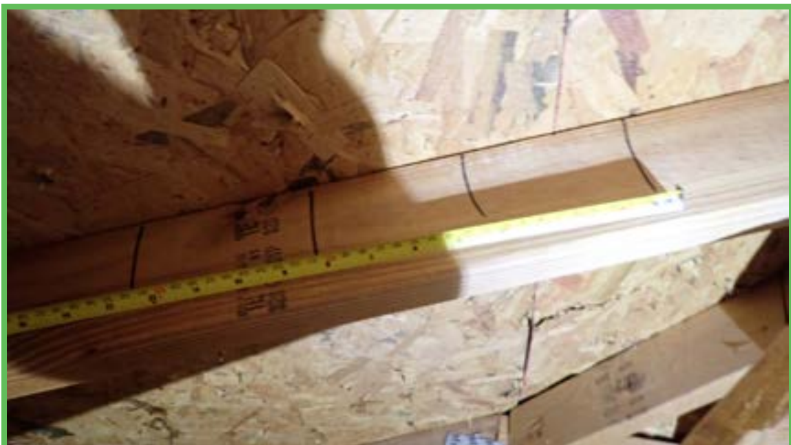
Roof Deck Attachment
