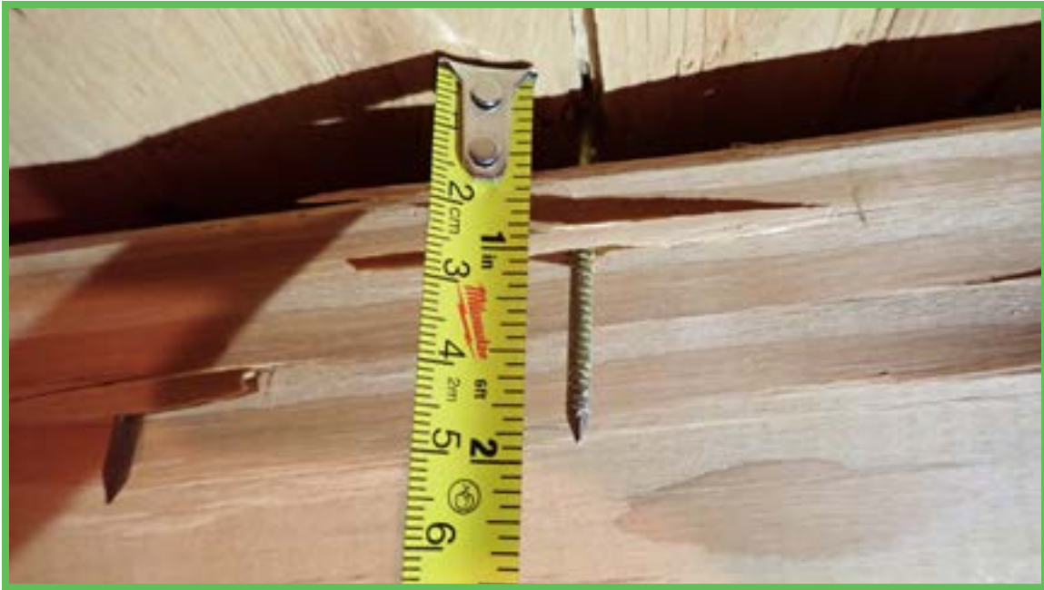
Roof Deck Attachment
