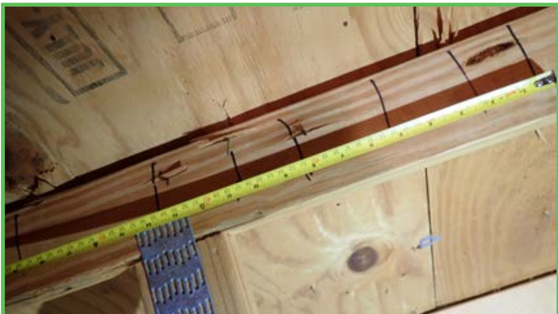
Roof Deck Attachment
