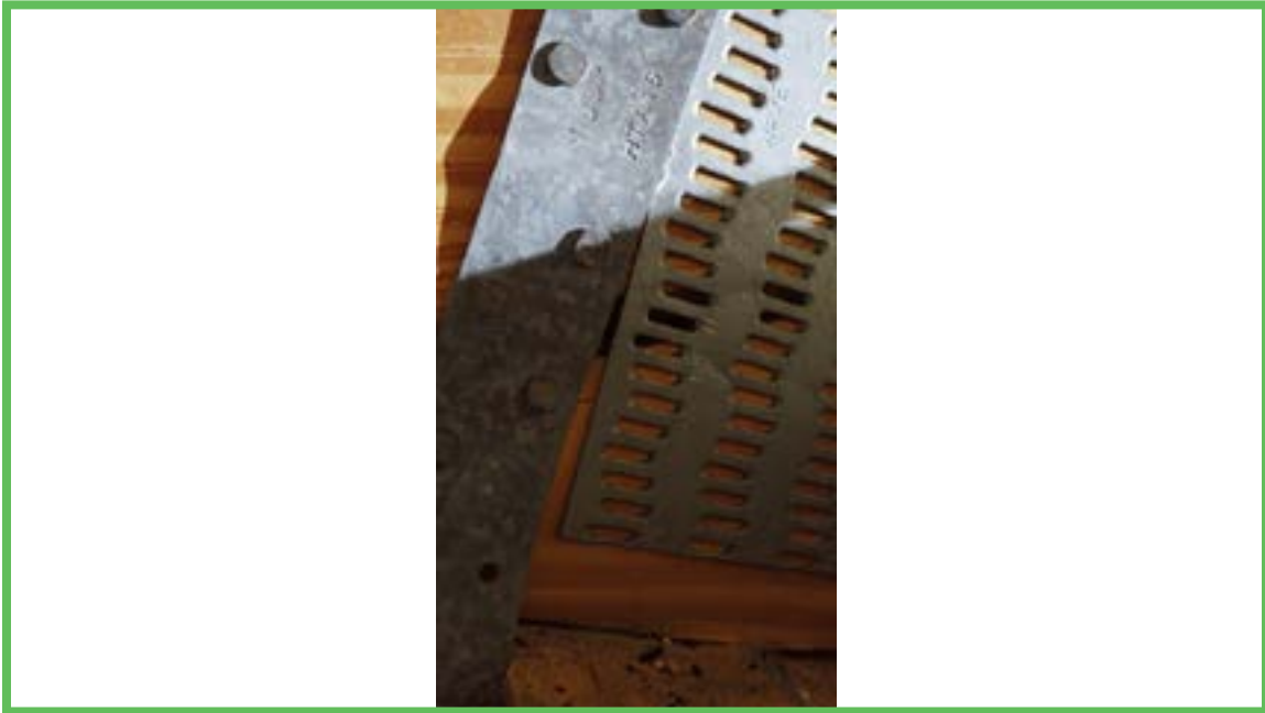
Roof to Wall Attachment
