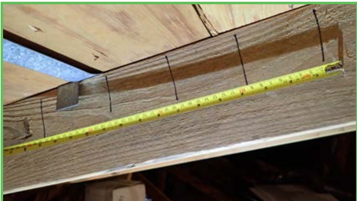
Roof Deck Attachment
