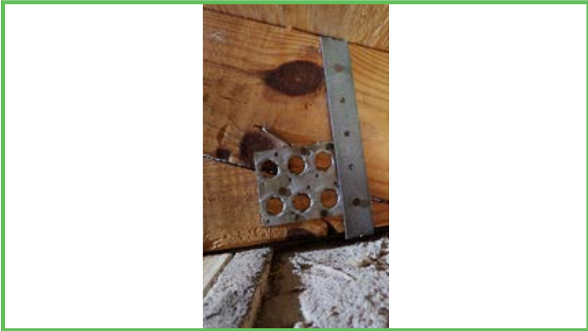
Roof to Wall Attachment
