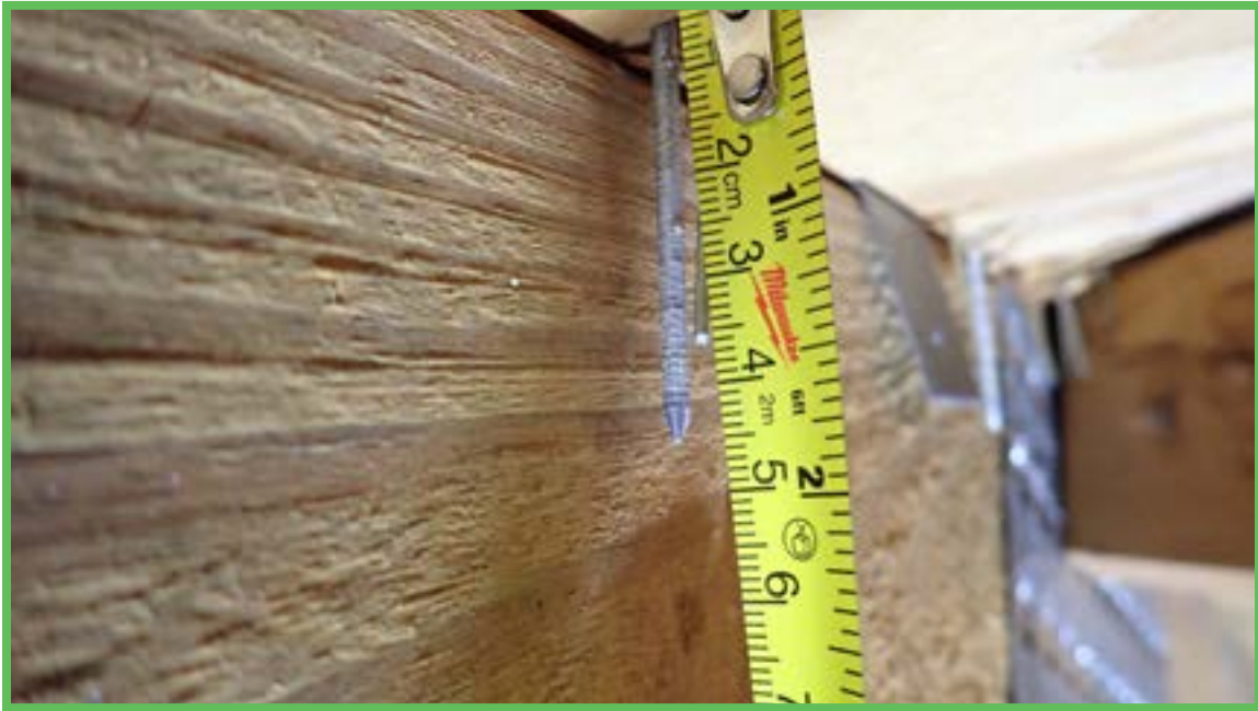
Roof Deck Attachment
