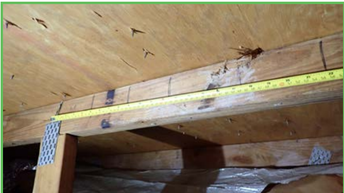
Roof Deck Attachment
