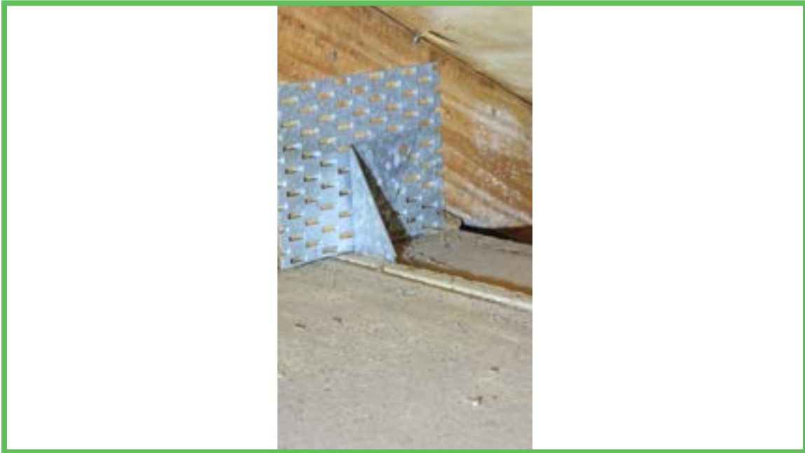
Roof to Wall Attachment
