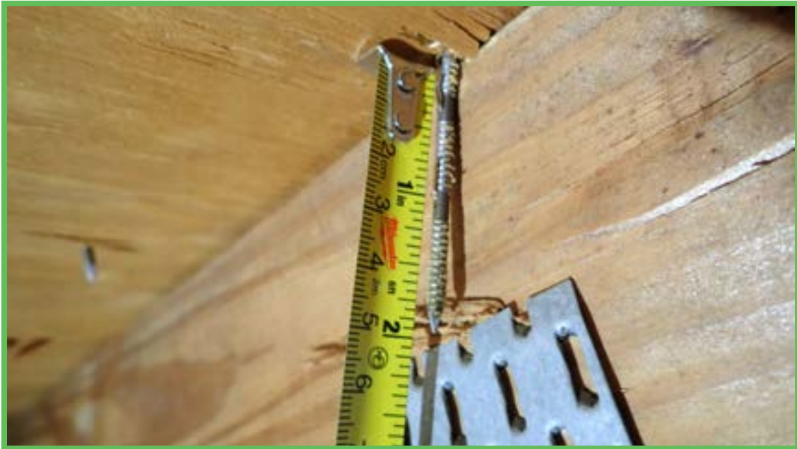
Roof Deck Attachment
