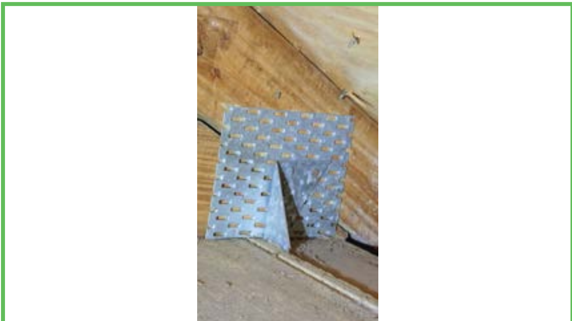
Roof to Wall Attachment
