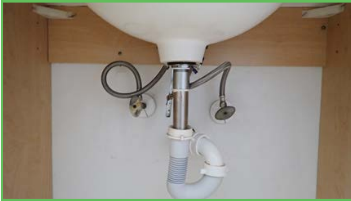
Under Sink1 Bath 2
