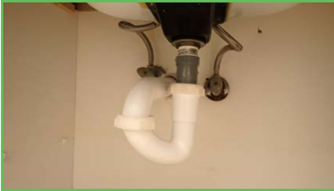
Under Sink1 Bath 1
