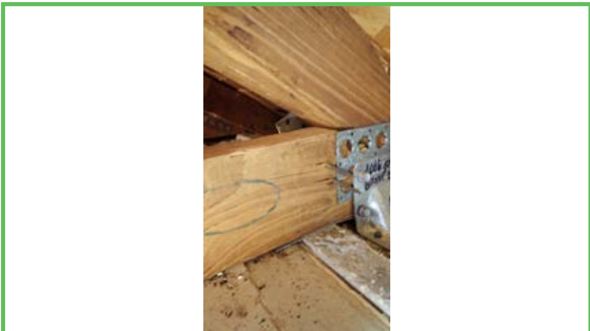
Roof to Wall Attachment
