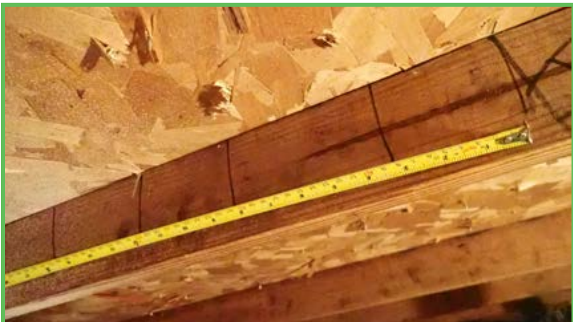
Roof Deck Attachment
