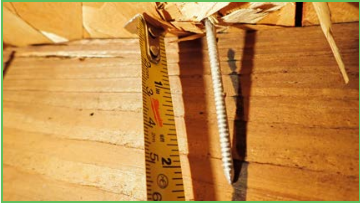
Roof Deck Attachment
