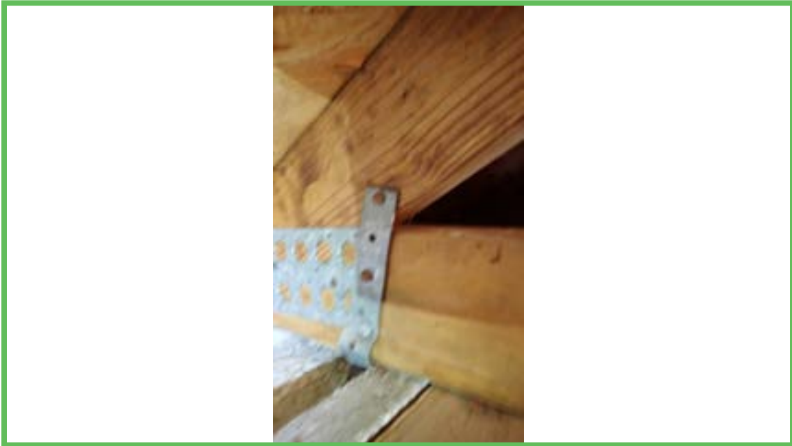
Roof to Wall Attachment
