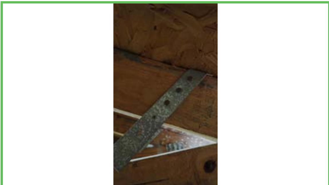
Roof to Wall Attachment
