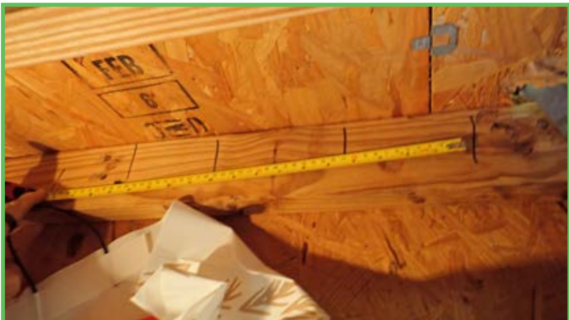
Roof Deck Attachment
