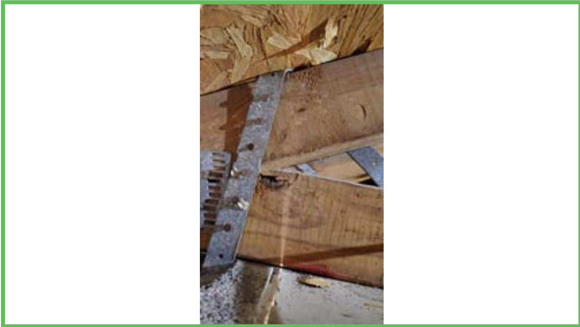
Roof to Wall Attachment
