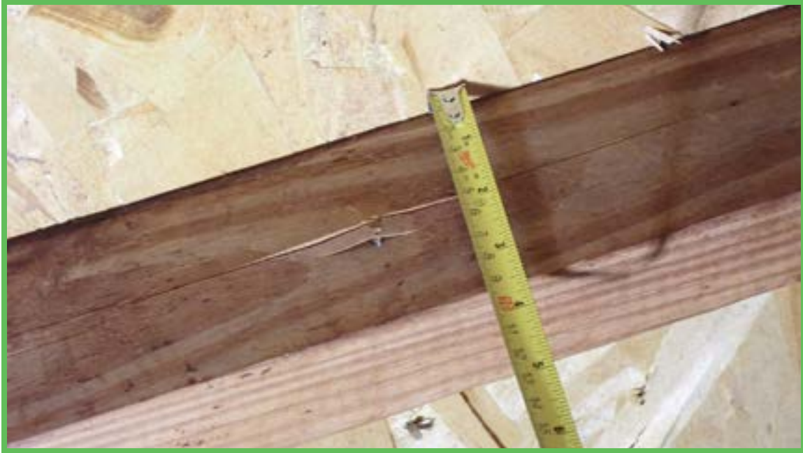
Roof Deck Attachment
