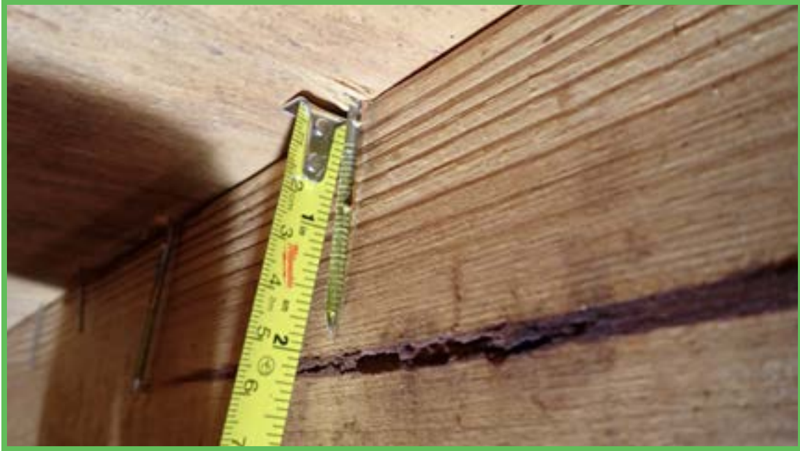
Roof Deck Attachment
