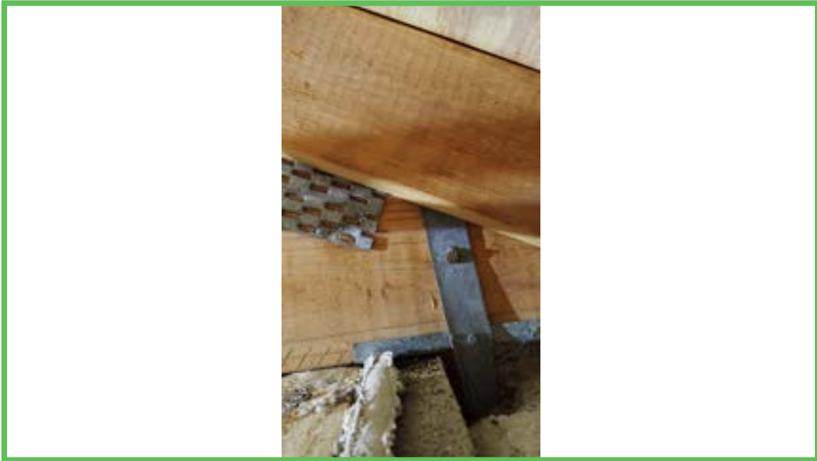
Roof to Wall Attachment
