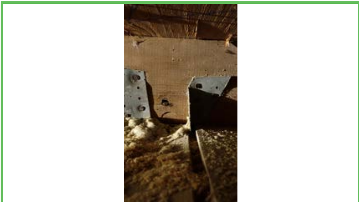
Roof to Wall Attachment
