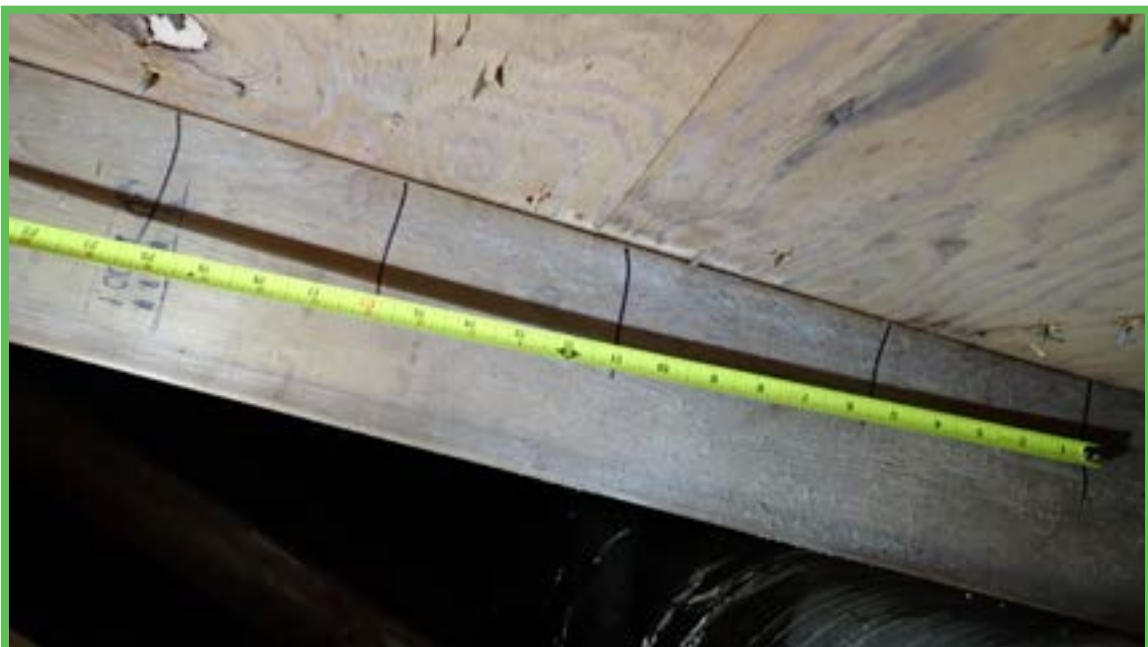
Roof Deck Attachment
