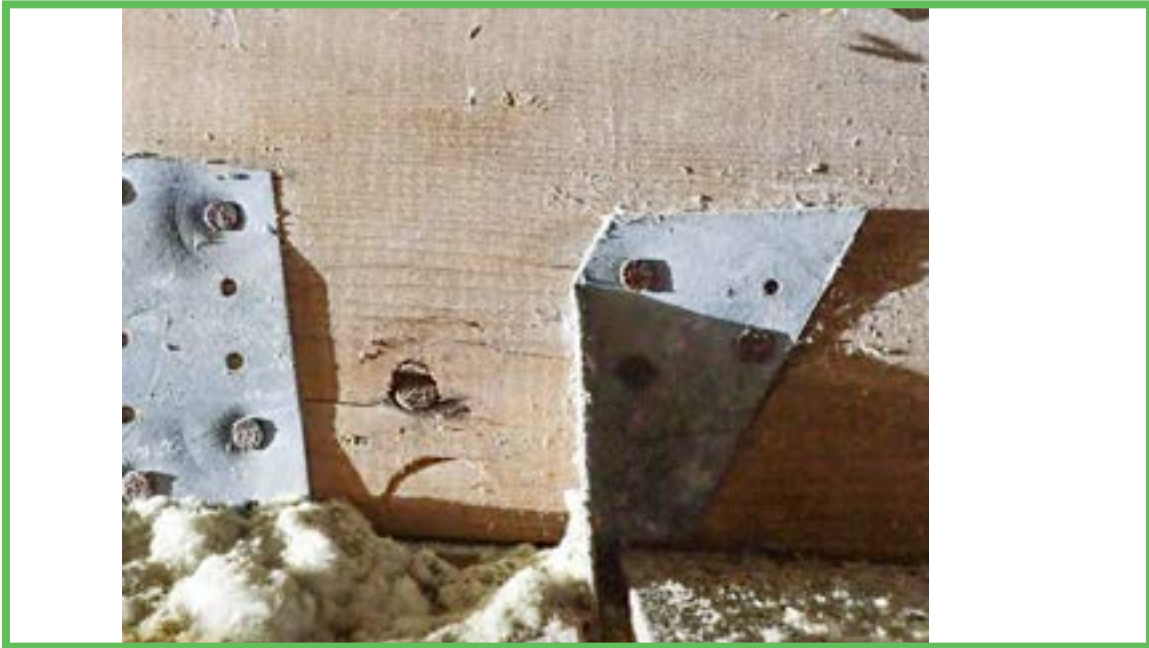
Roof to Wall Attachment
