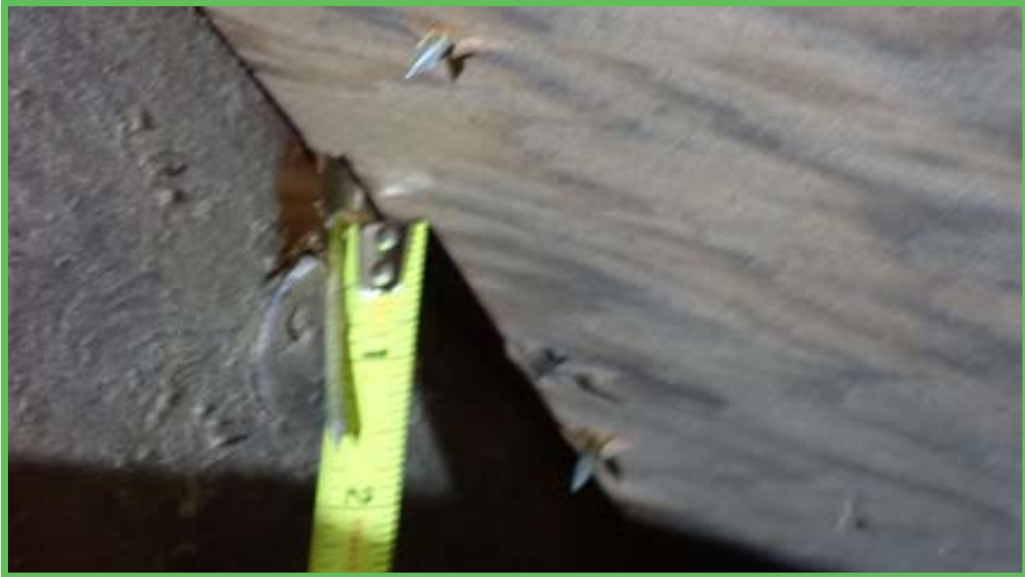
Roof Deck Attachment
