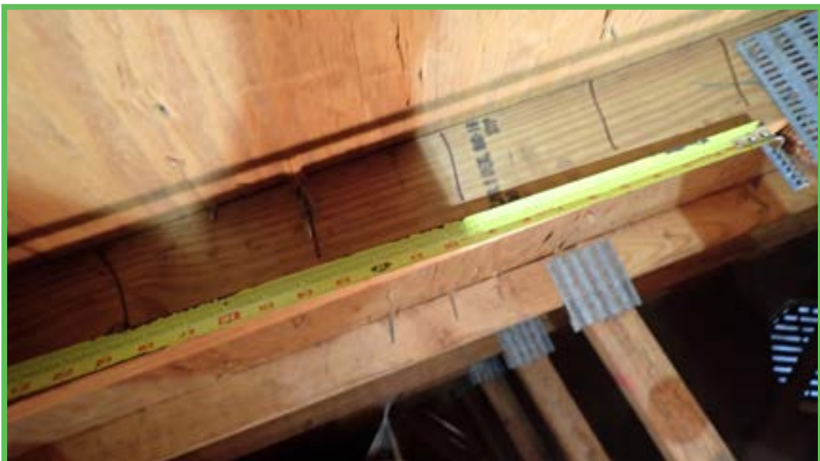
Roof Deck Attachment
