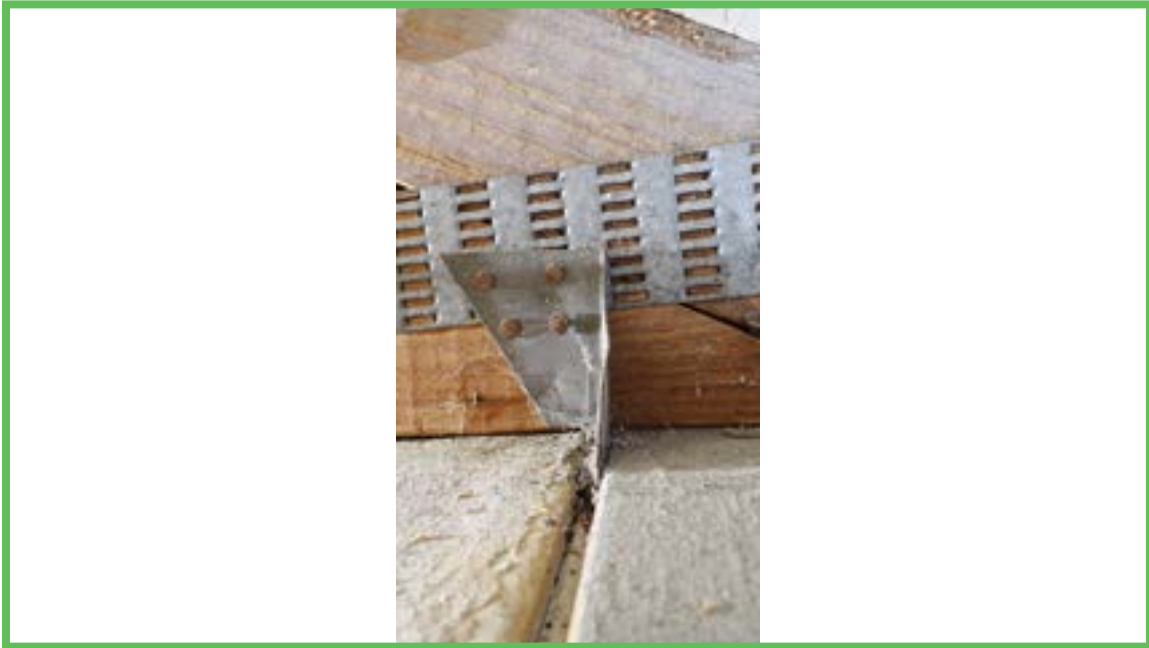
Roof to Wall Attachment
