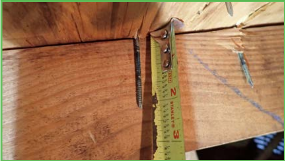
Roof Deck Attachment
