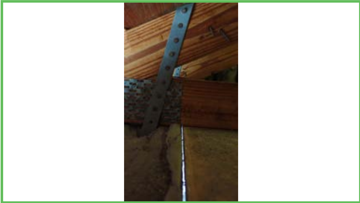
Roof to Wall Attachment
