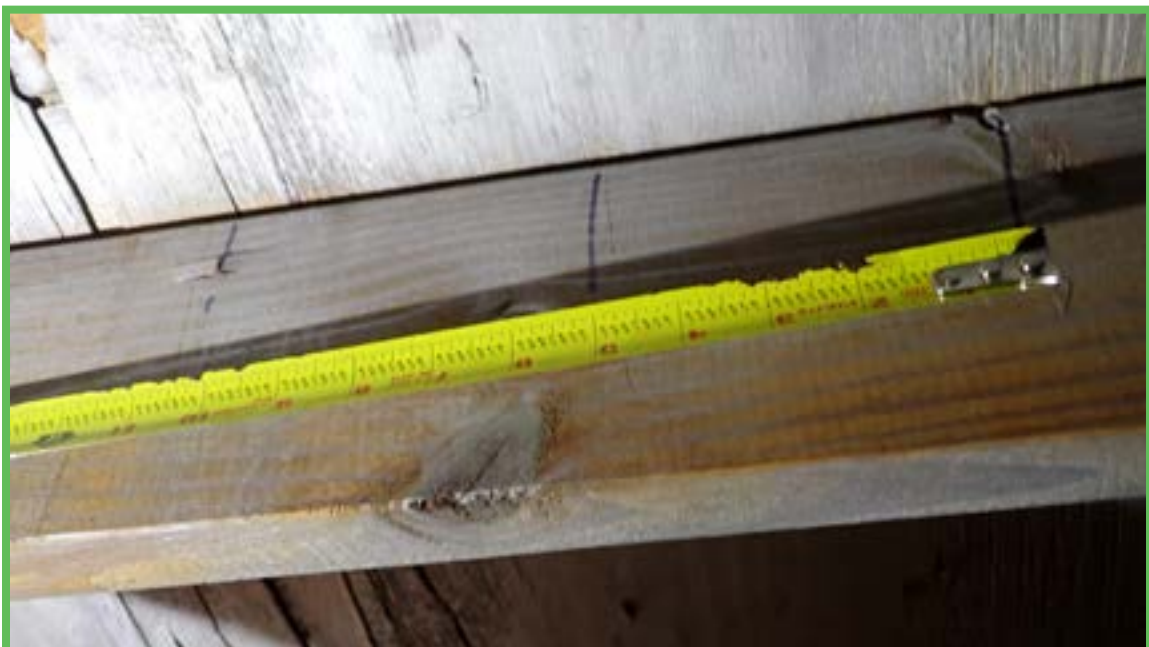
Roof Deck Attachment
