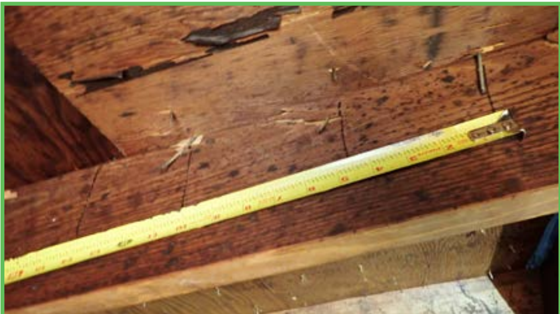
Roof Deck Attachment
