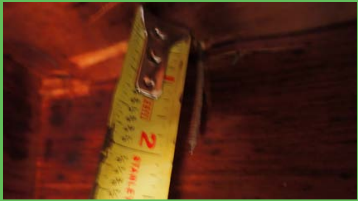
Roof Deck Attachment
