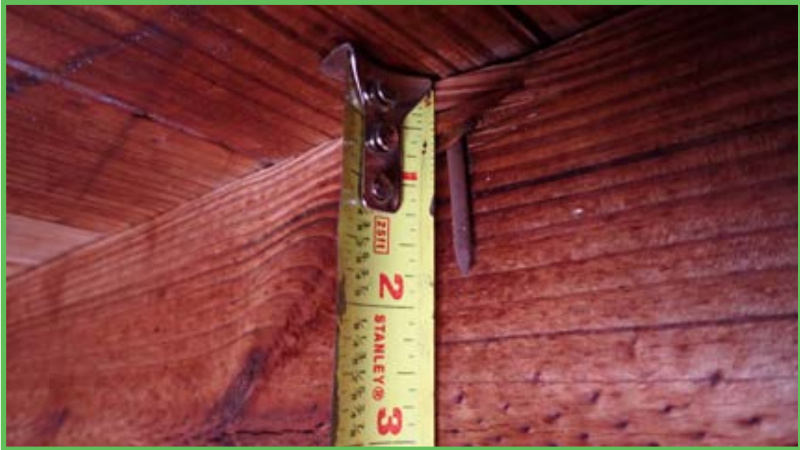
Roof Deck Attachment
