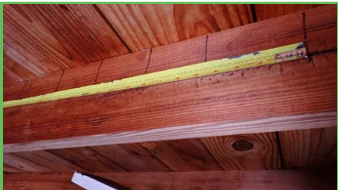
Roof Deck Attachment
