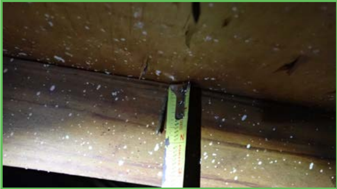
Roof Deck Attachment
