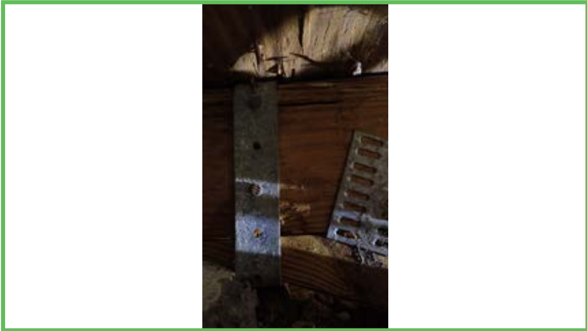
Roof to Wall Attachment
