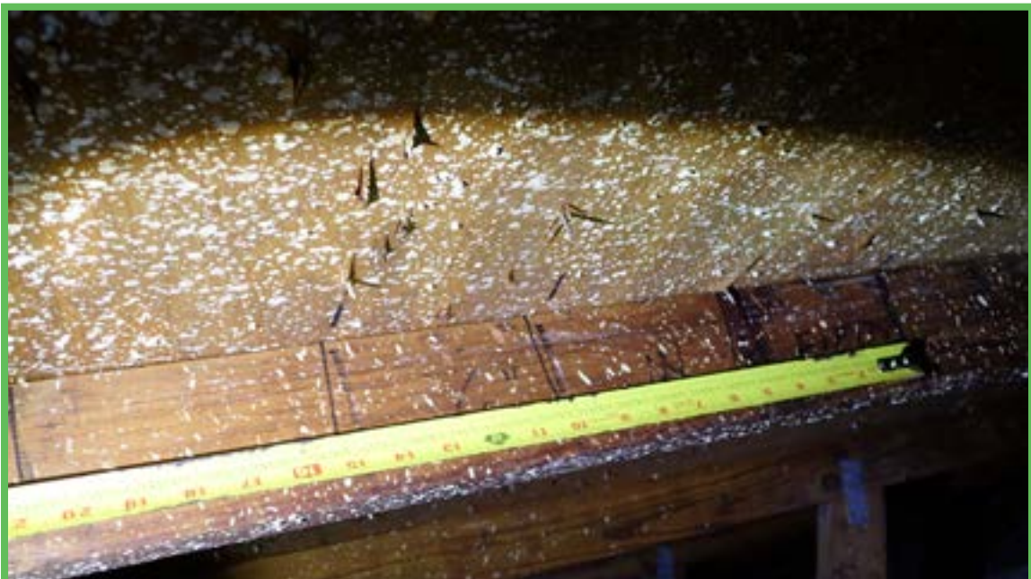
Roof Deck Attachment
