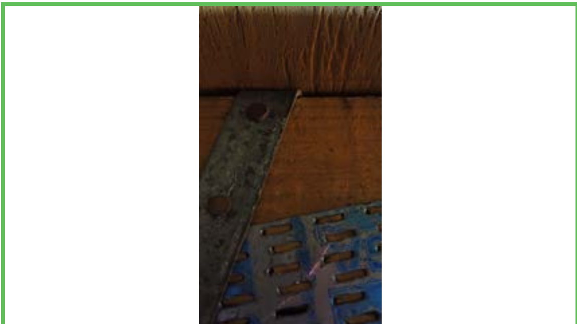
Roof to Wall Attachment
