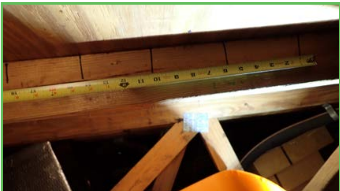
Roof Deck Attachment
