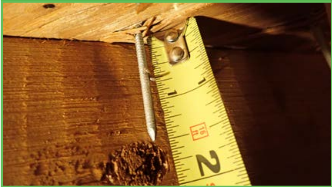
Roof Deck Attachment
