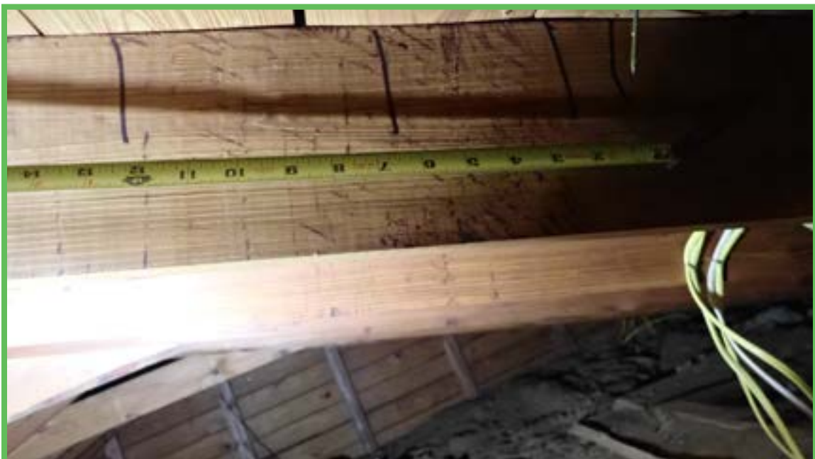
Roof Deck Attachment
