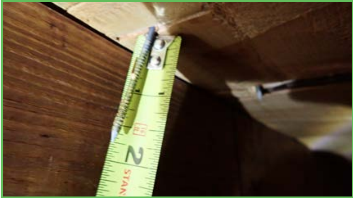
Roof Deck Attachment
