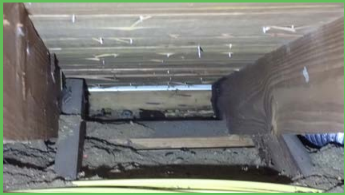
Roof to Wall Attachment
