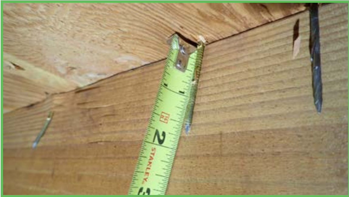
Roof Deck Attachment
