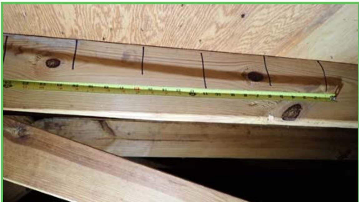
Roof Deck Attachment
