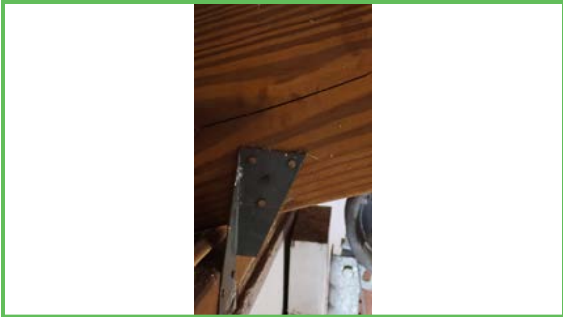
Roof to Wall Attachment
