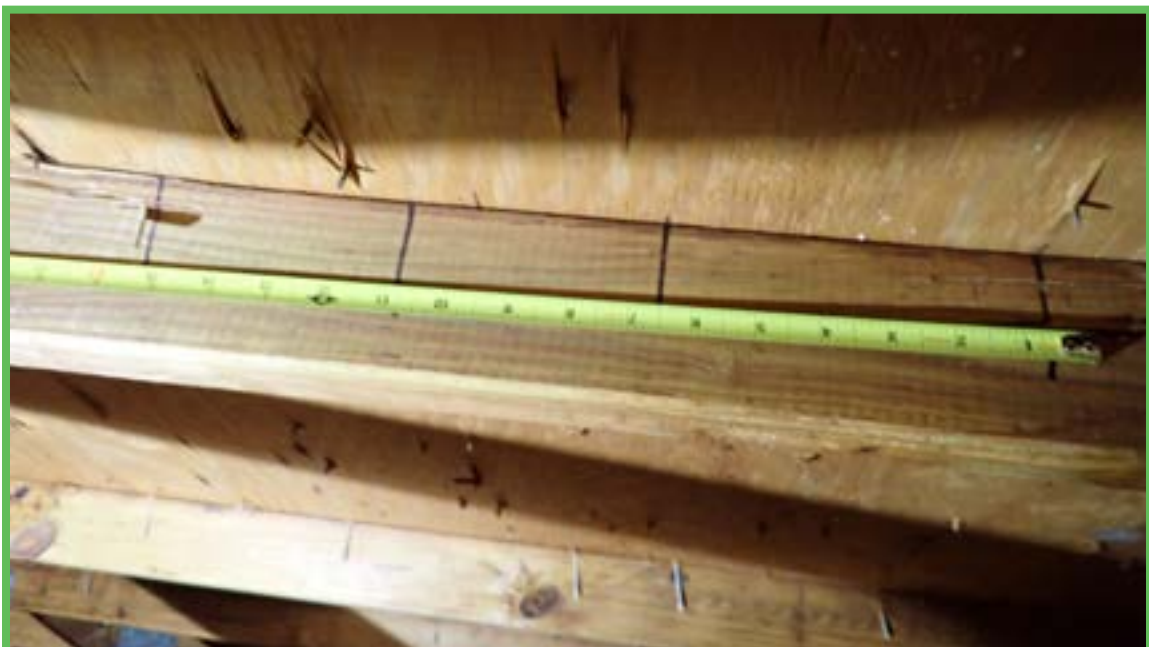
Roof Deck Attachment
