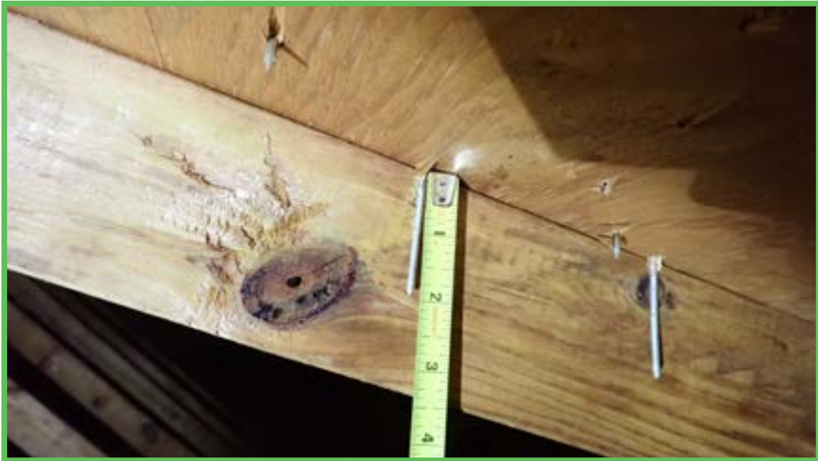
Roof Deck Attachment
