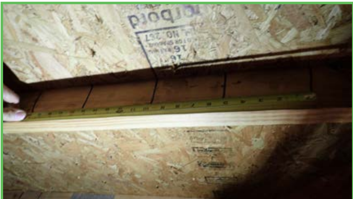
Roof Deck Attachment
