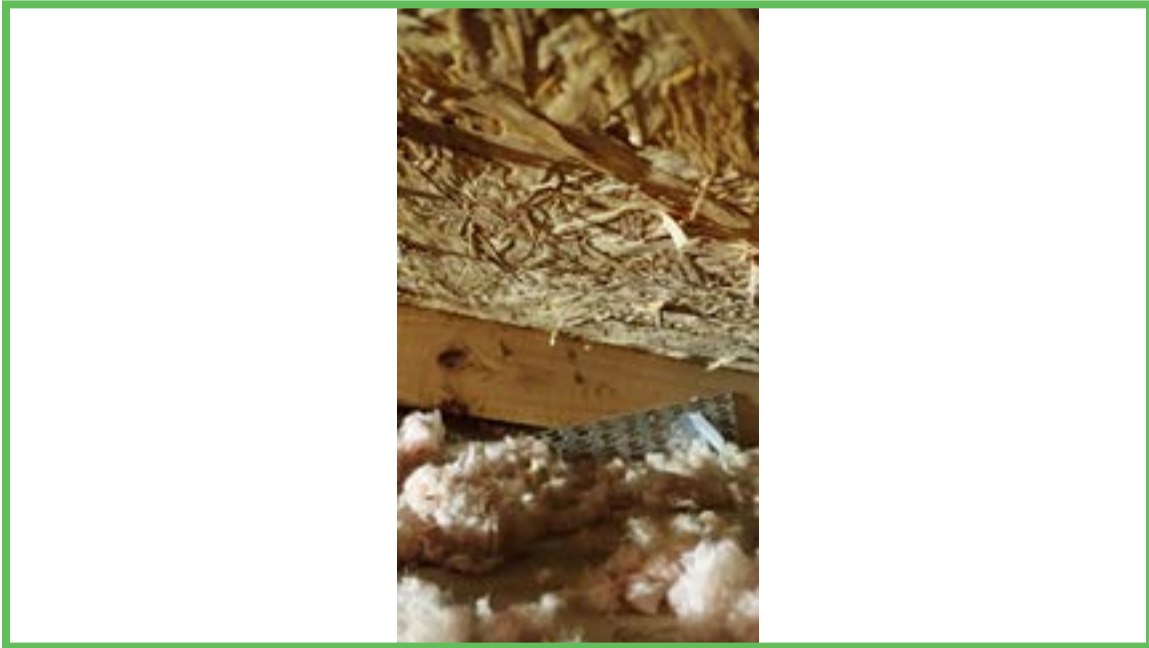
Roof to Wall Attachment
