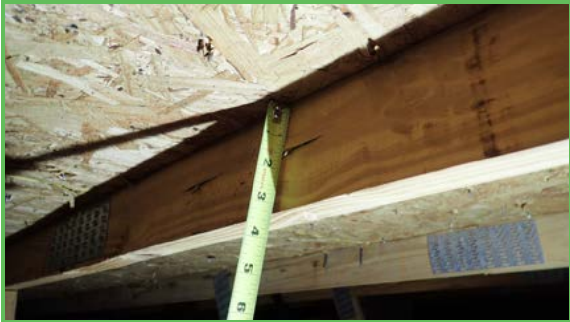
Roof Deck Attachment
