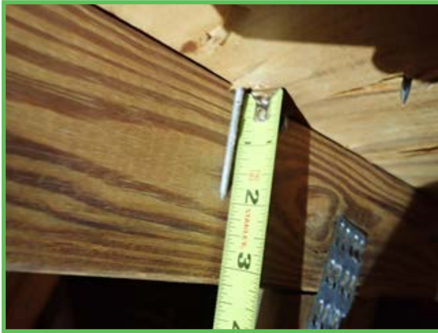
Roof Deck Attachment
