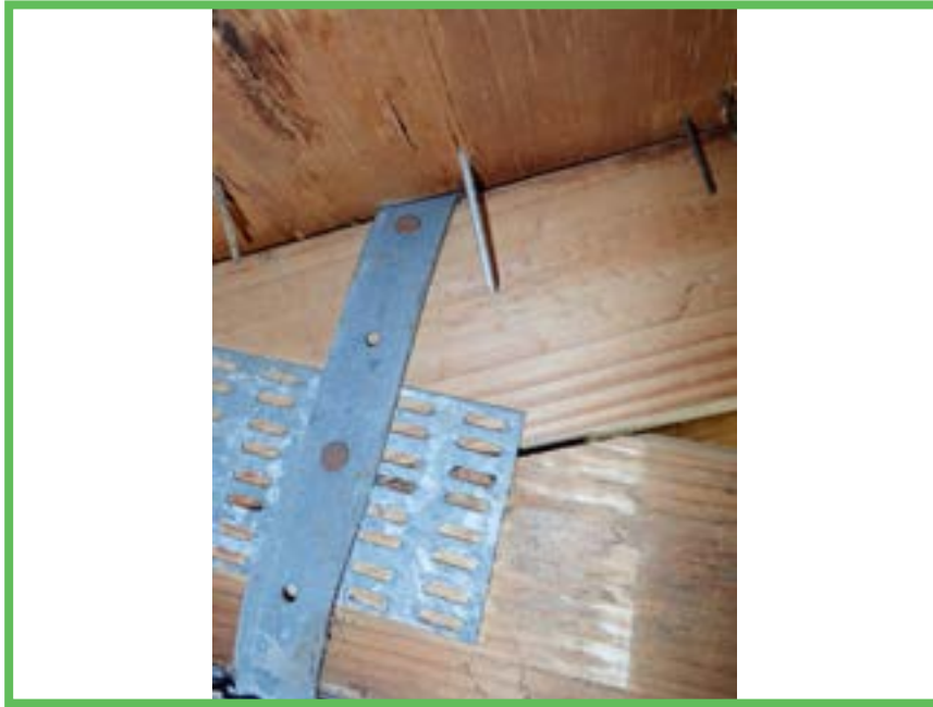
Roof to Wall Attachment
