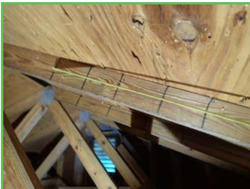
Roof Deck Attachment
