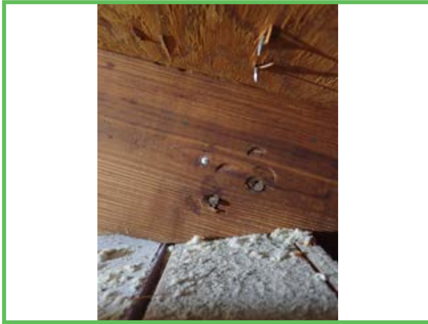
Roof to Wall Attachment
