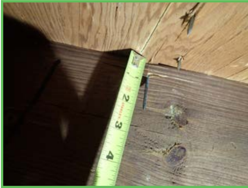
Roof Deck Attachment
