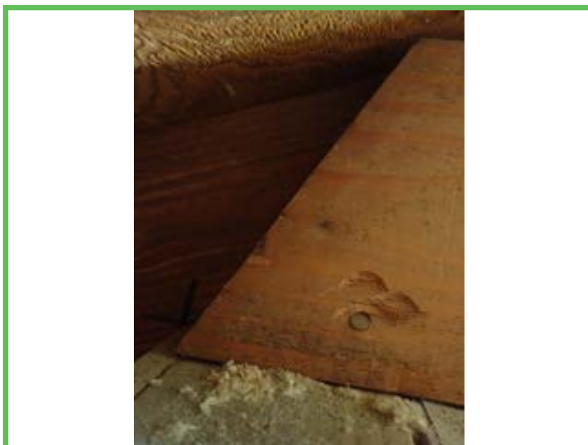
Roof to Wall Attachment
