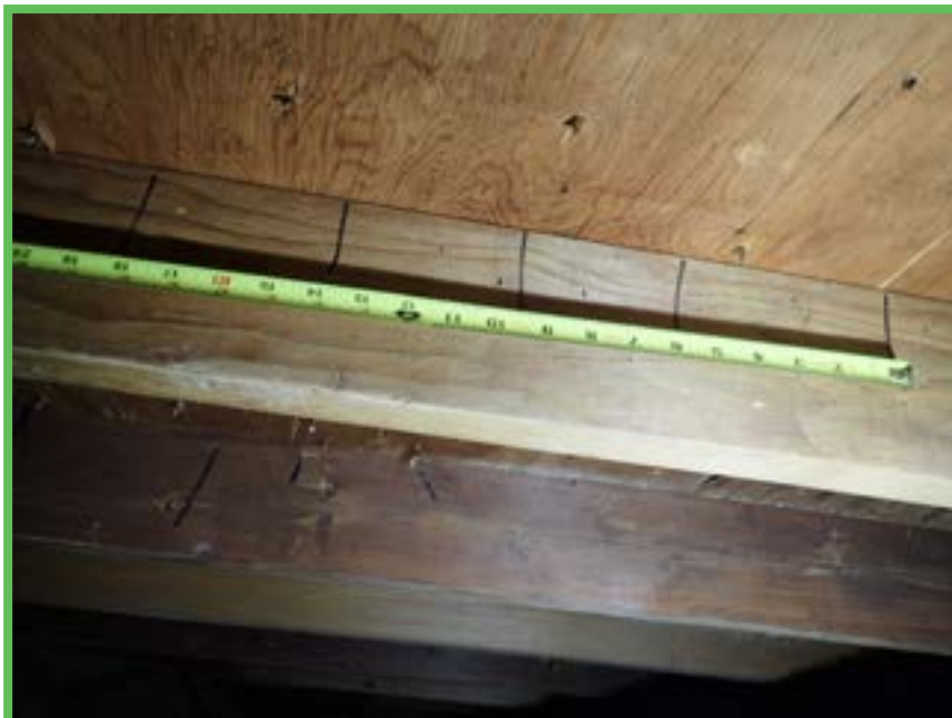
Roof Deck Attachment
